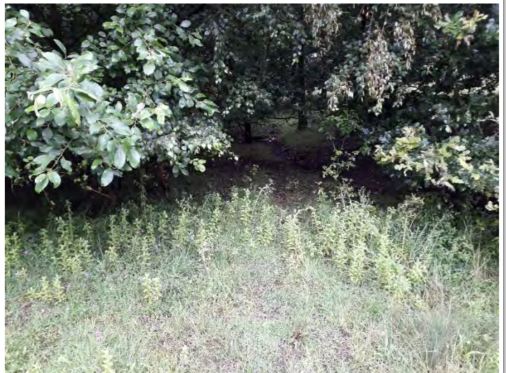
Existing ditch leading to possible soakaway chamber
