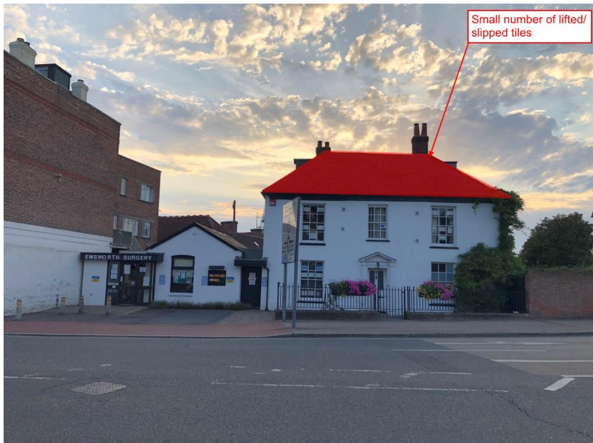
Image 4.3.3 Location of potential bat access points and potential roost locations on the east elevation of the building.
