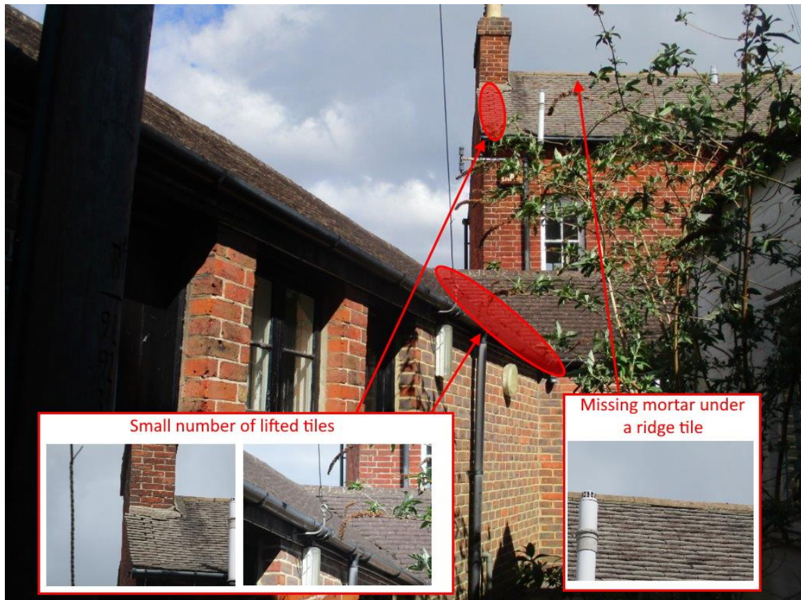
Image 4.3.4 Location of potential bat access points and potential roost locations on the south elevation of the building and within the courtyard.
