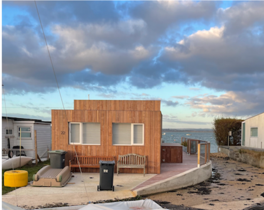
Photo 4: new locker looking north. Its height sits just below the window level.
