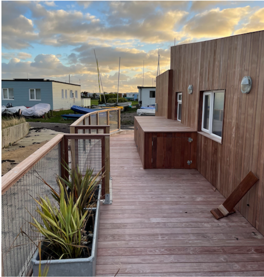
Photo 6: New locker looking south shortly after completion. The new locker is the same height and roughly the same dimensions as the original but positioned slightly further south to enable the steps to the slip to be safely fenced off with protective fencing.
