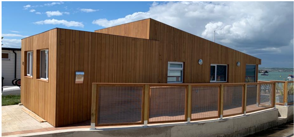
Photo 5: New locker looking west shortly after completion. The new locker is the same height and roughly the same dimensions as the original but positioned further south to enable the steps to the slip to be safely fenced off with protective fencing.
