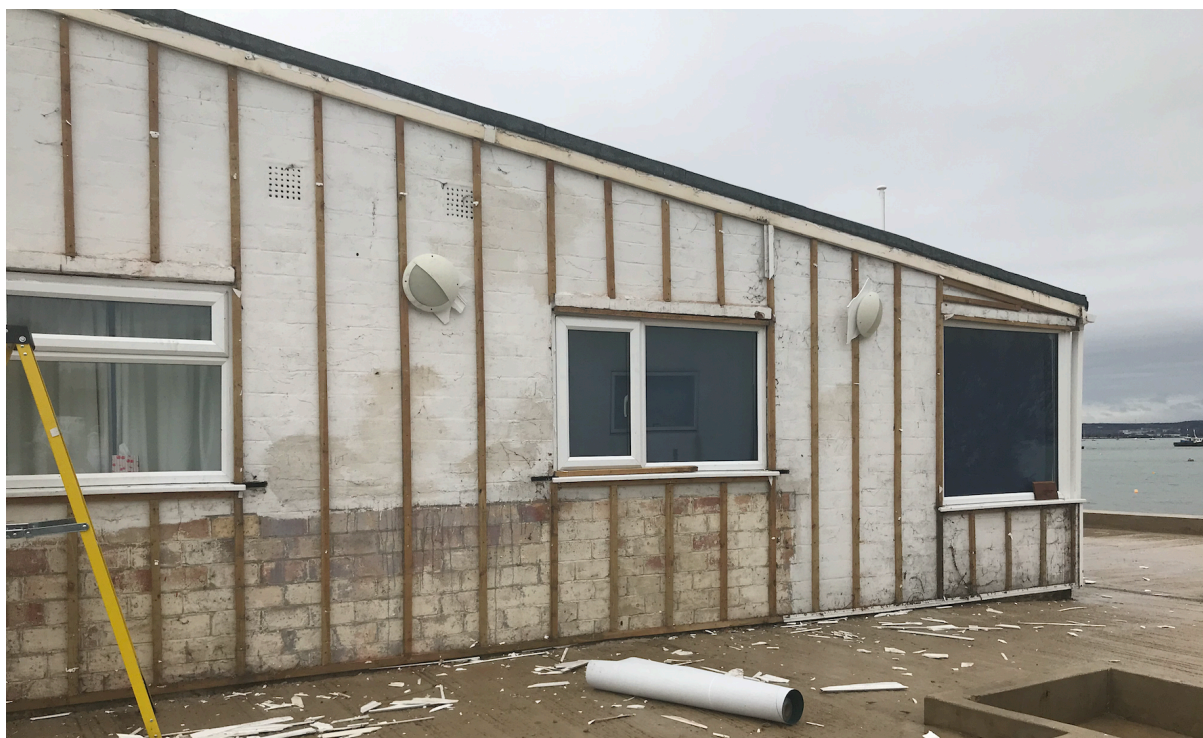
Photo 2: East evaluation. The unpainted area beneath the window shows the extent of the original locker in terms of height and length.
