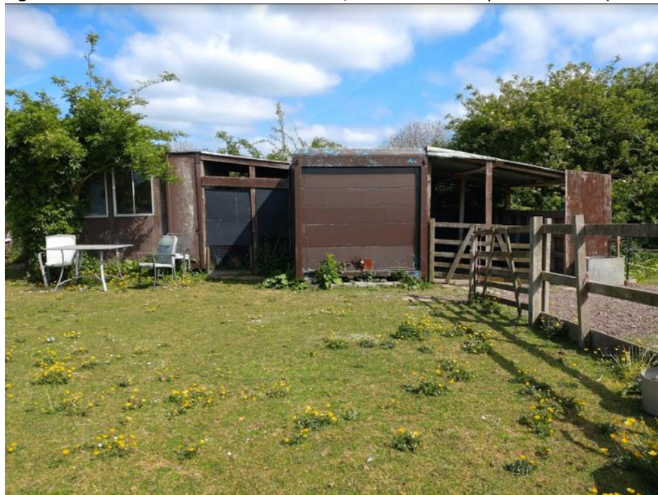
Figure 11. View of one of several horse stable/shelter structures present on-site (taken May, 2022).
