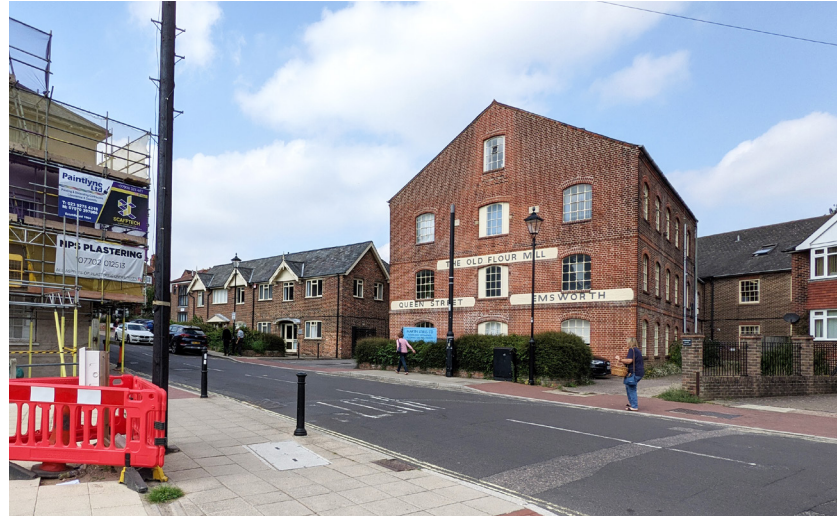
2.2 View from Site to Flour Mill.
