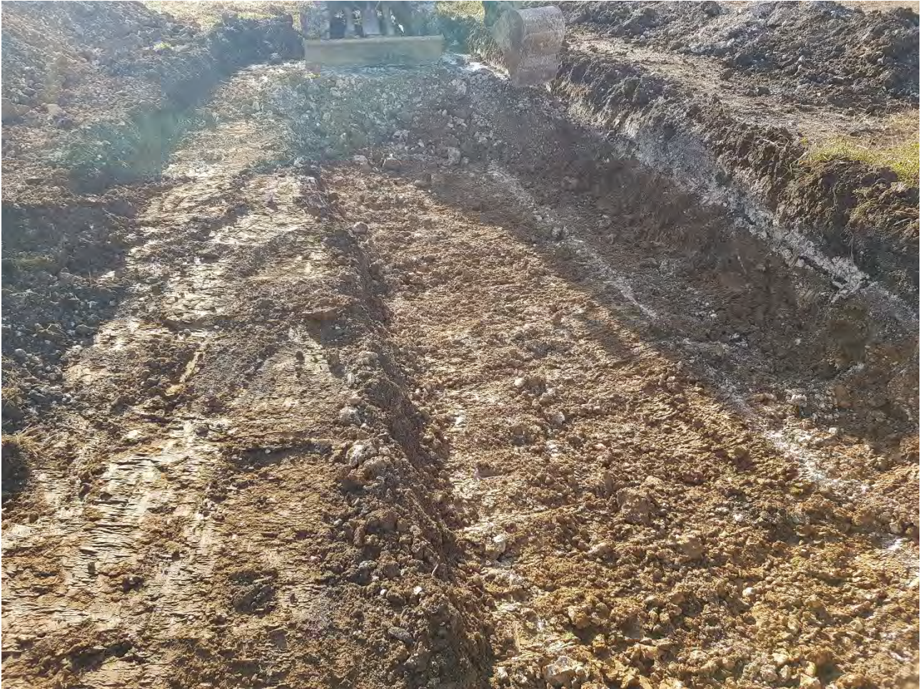
Plate 17 – View south across excavation
