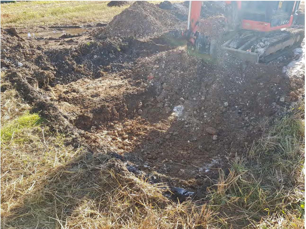
Plate 14 – View of excavation being deepened to removed full depth of Made Ground
