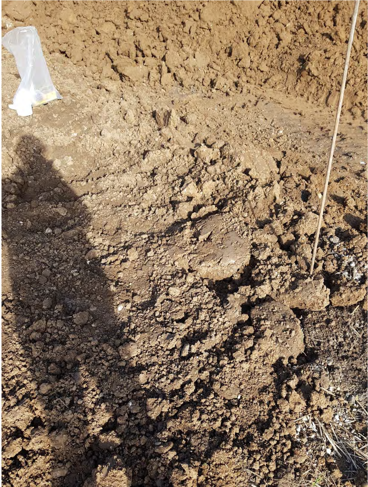
Plate 2 – Topsoil placed in excavation
