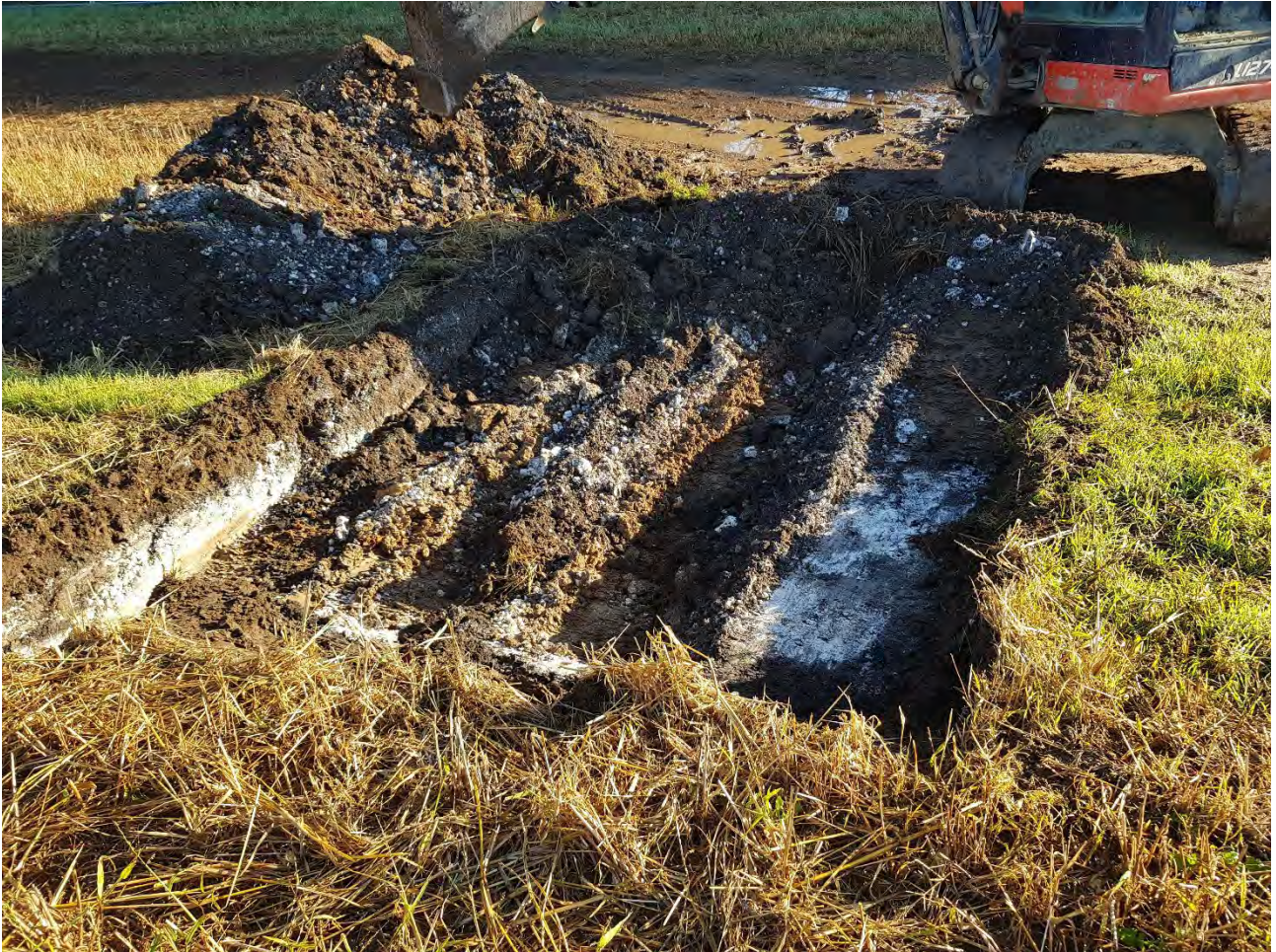
Plate 6 – Excavation in progress
