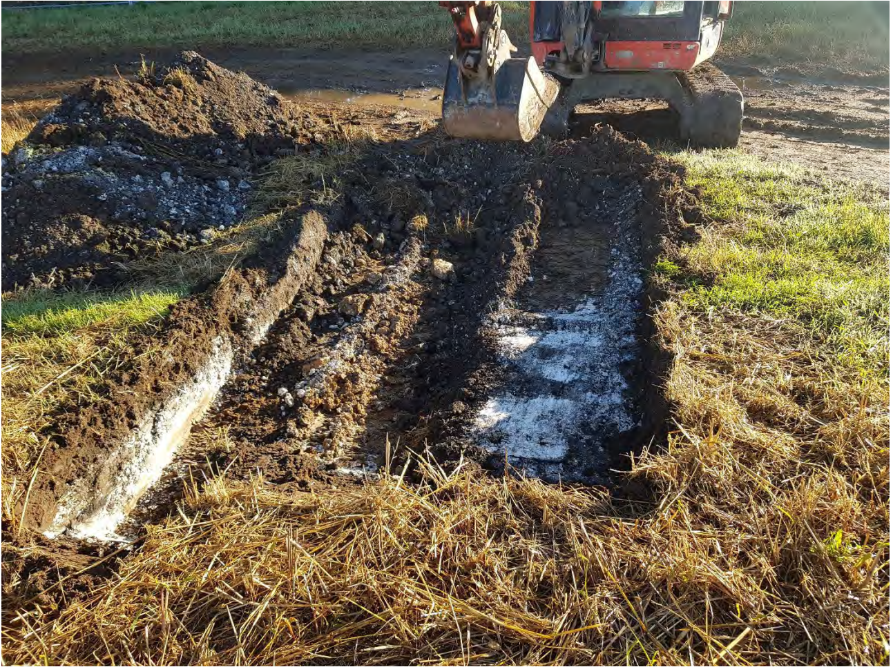
Plate 5 – View of north portion of excavation in progress
