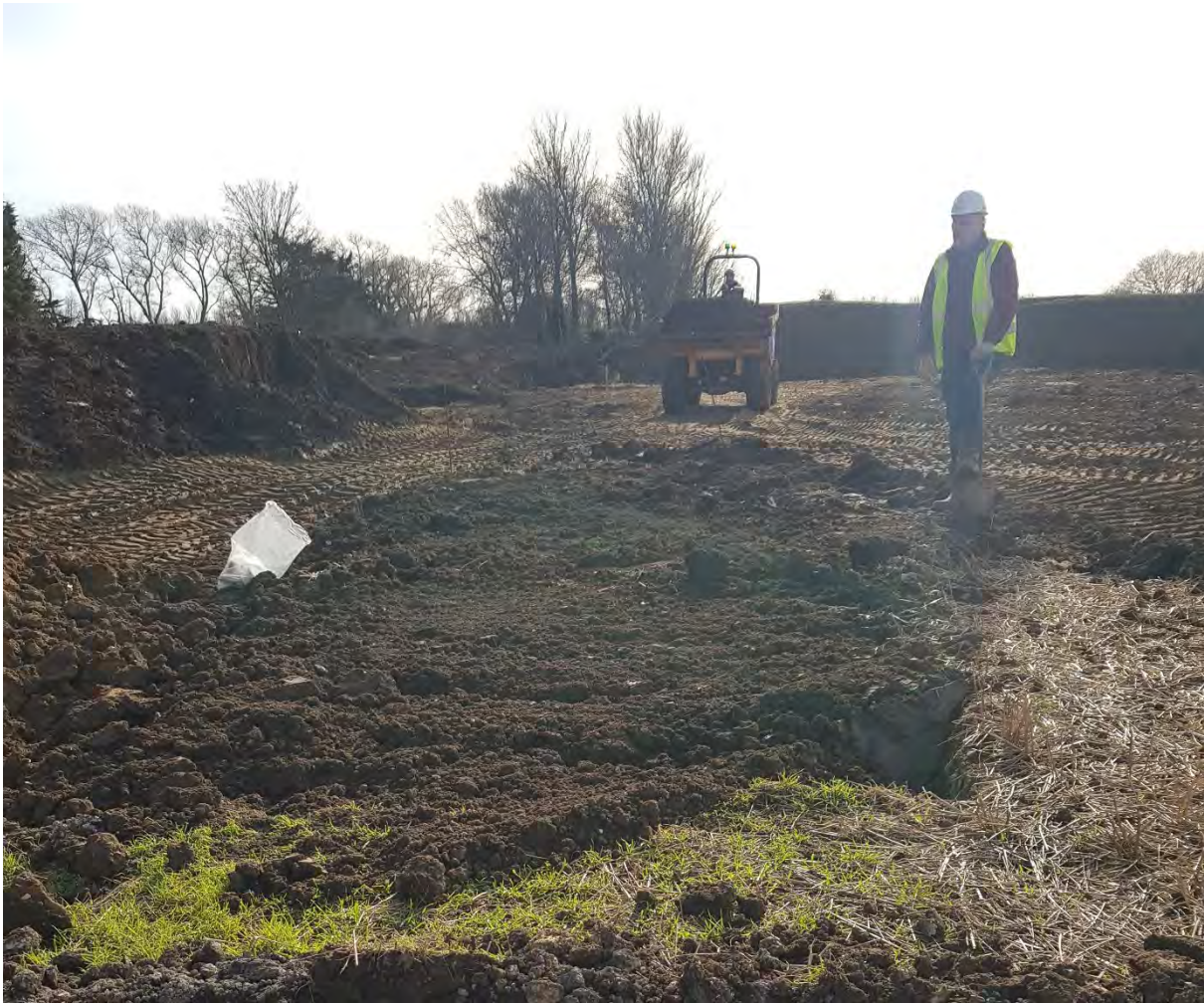
Plate 6 – View of backfilled excavation area
