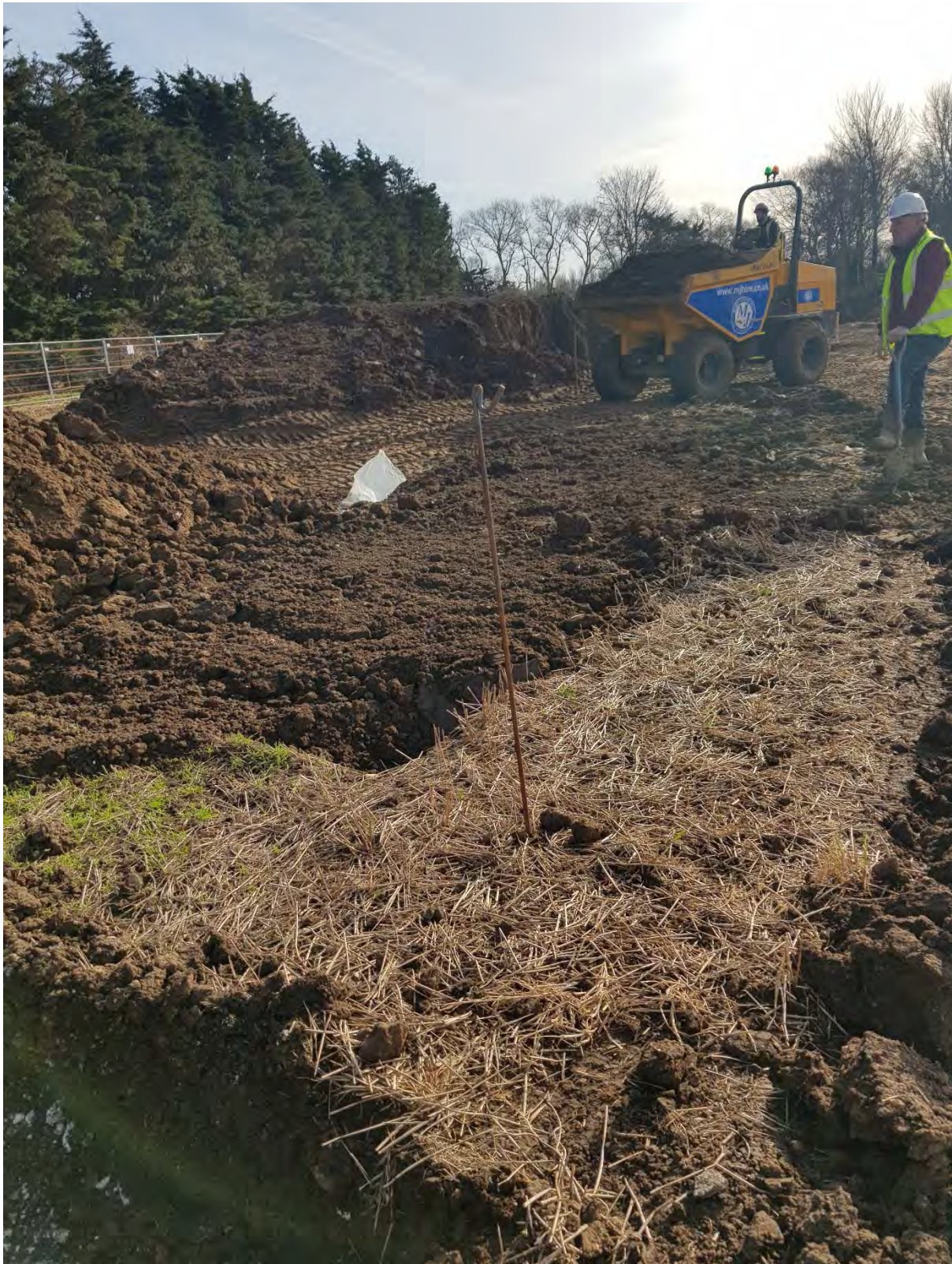
Plate 7 – View of backfilled excavation area
