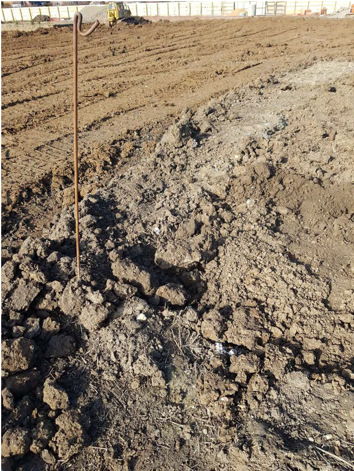
Plate 1 – Topsoil material placed in excavation
