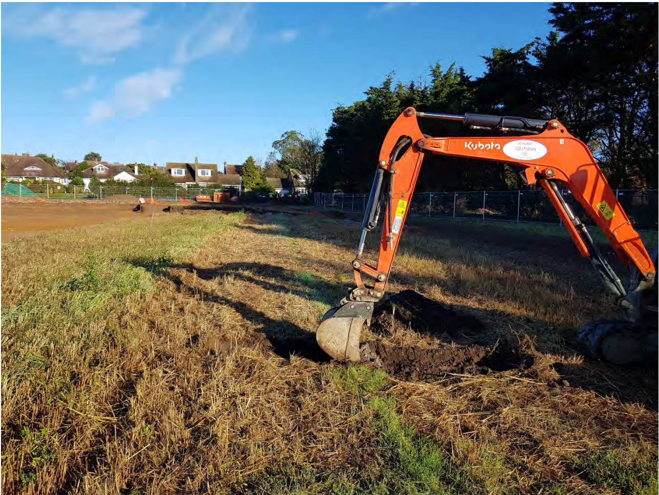
Plate 1 – View north showing the area of impacted ground to be excavated
