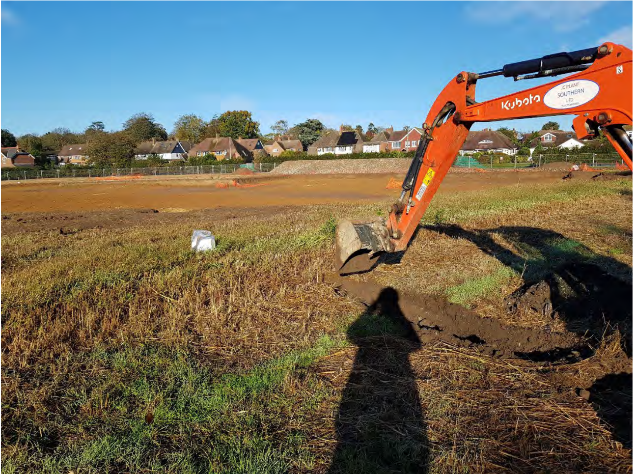
Plate 2 – View north west across the area to be excavated
