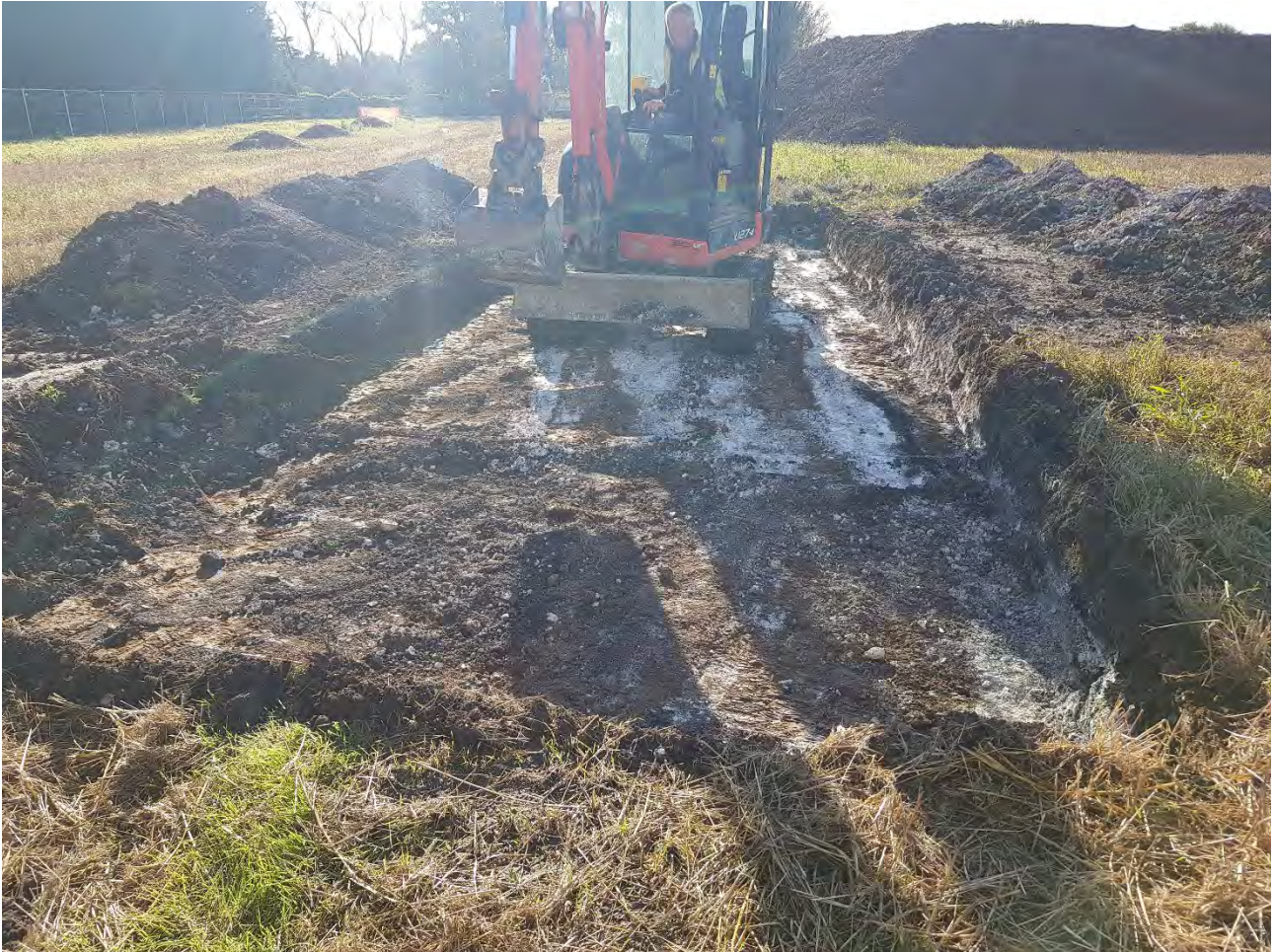
Plate 13 – View of excavation in progress, excavation being deepened to remove Made Ground
