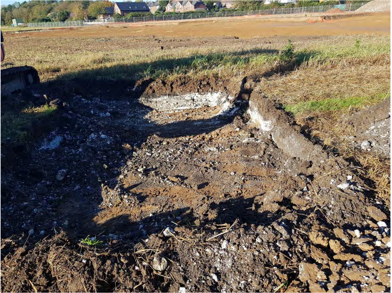
Plate 11 – View west across excavation
