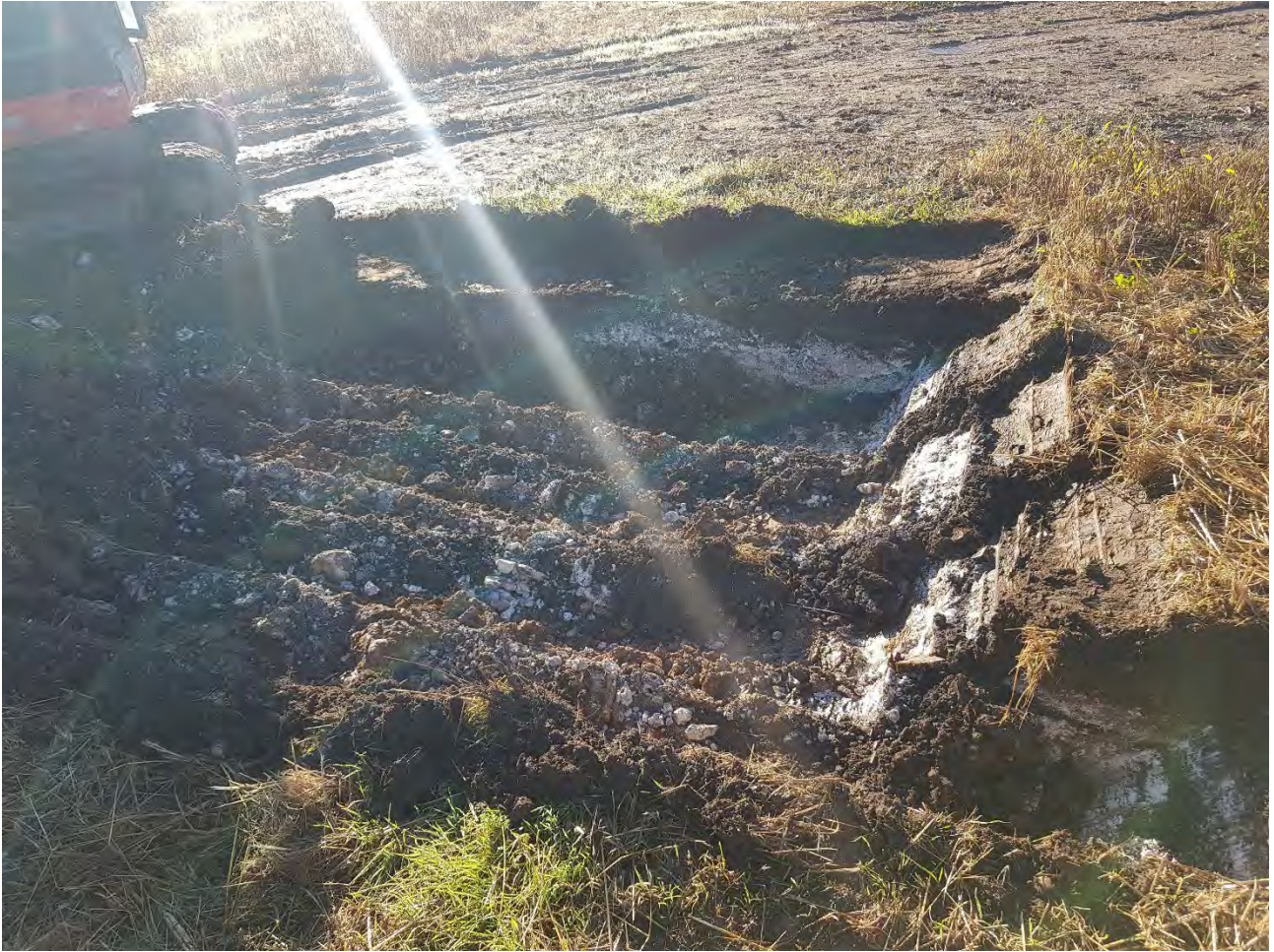
Plate 7 – Excavation being taken across the width of the farm track
