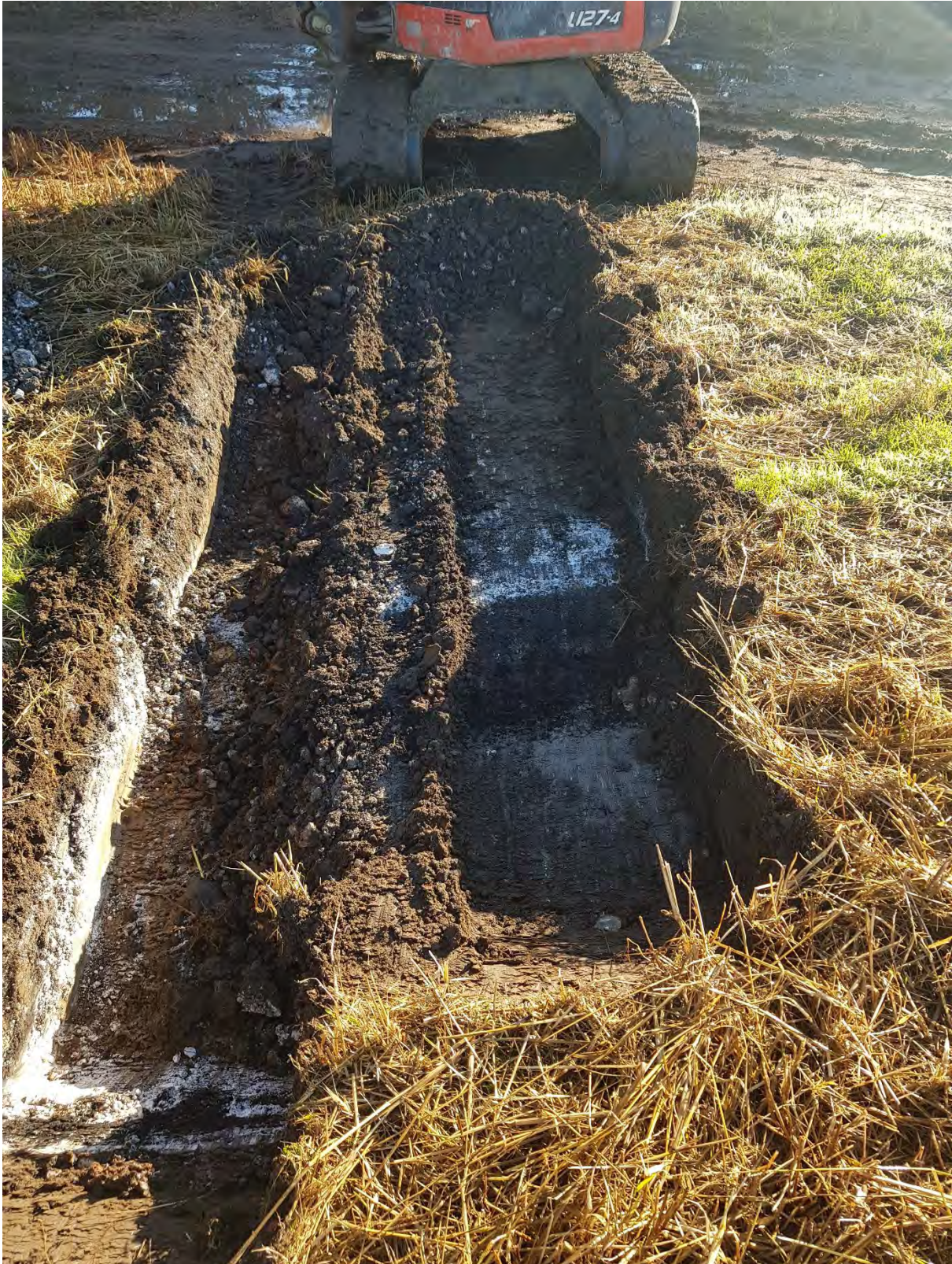
Plate 4 – Excavation in progress showing Made Ground materials
