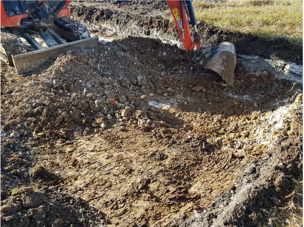
Plate 15 – View of natural soils exposed beneath the Made Ground materials
