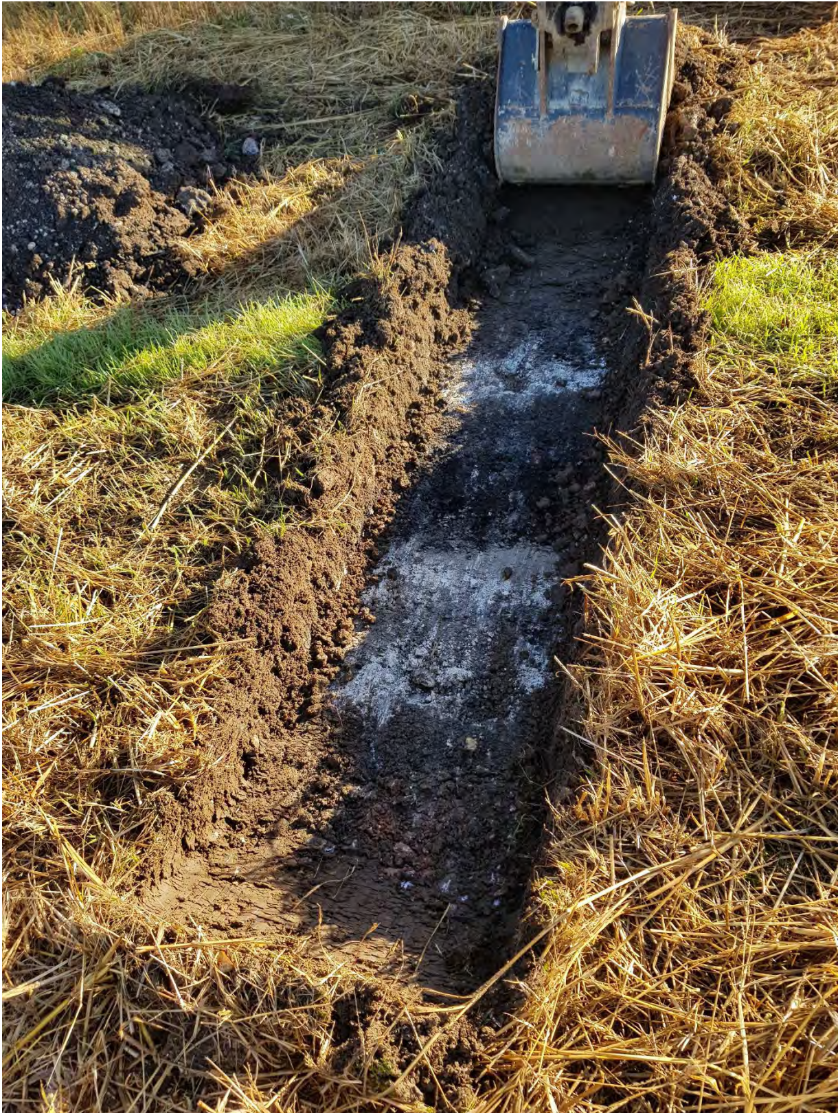
Plate 3 – View of the start of the excavation exposing Made Ground soils
