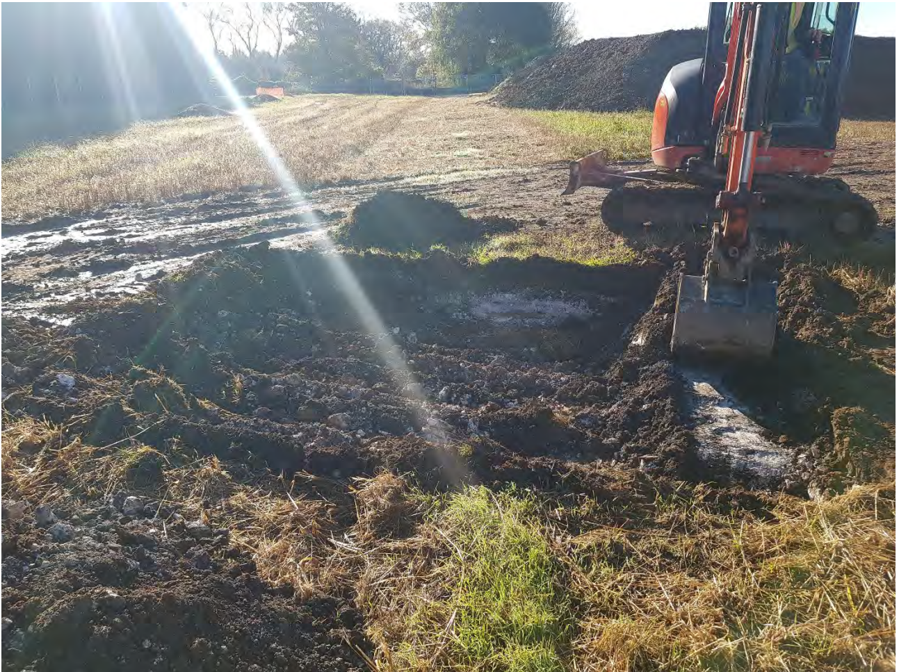
Plate 8 – Excavation being extended to full width of the farm track
