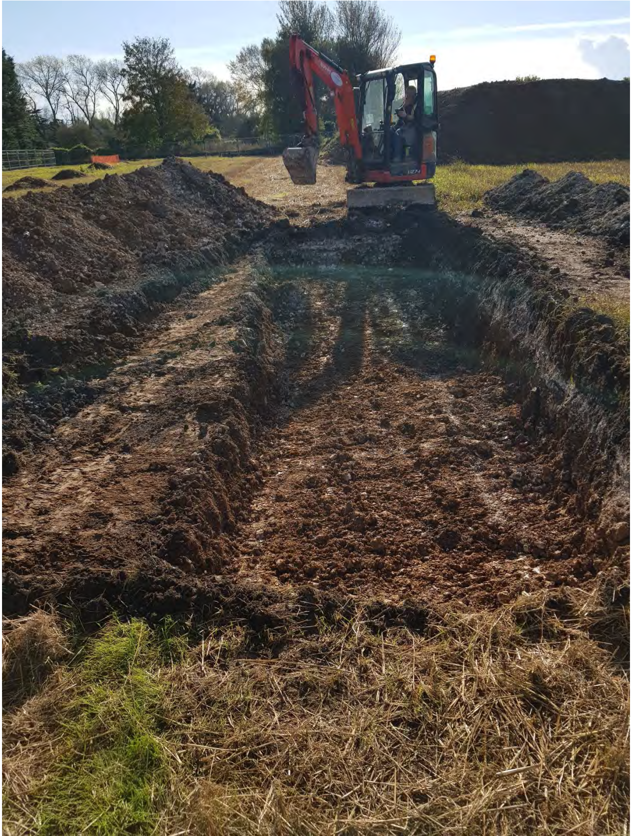
Plate 19 – View south across completed excavation
