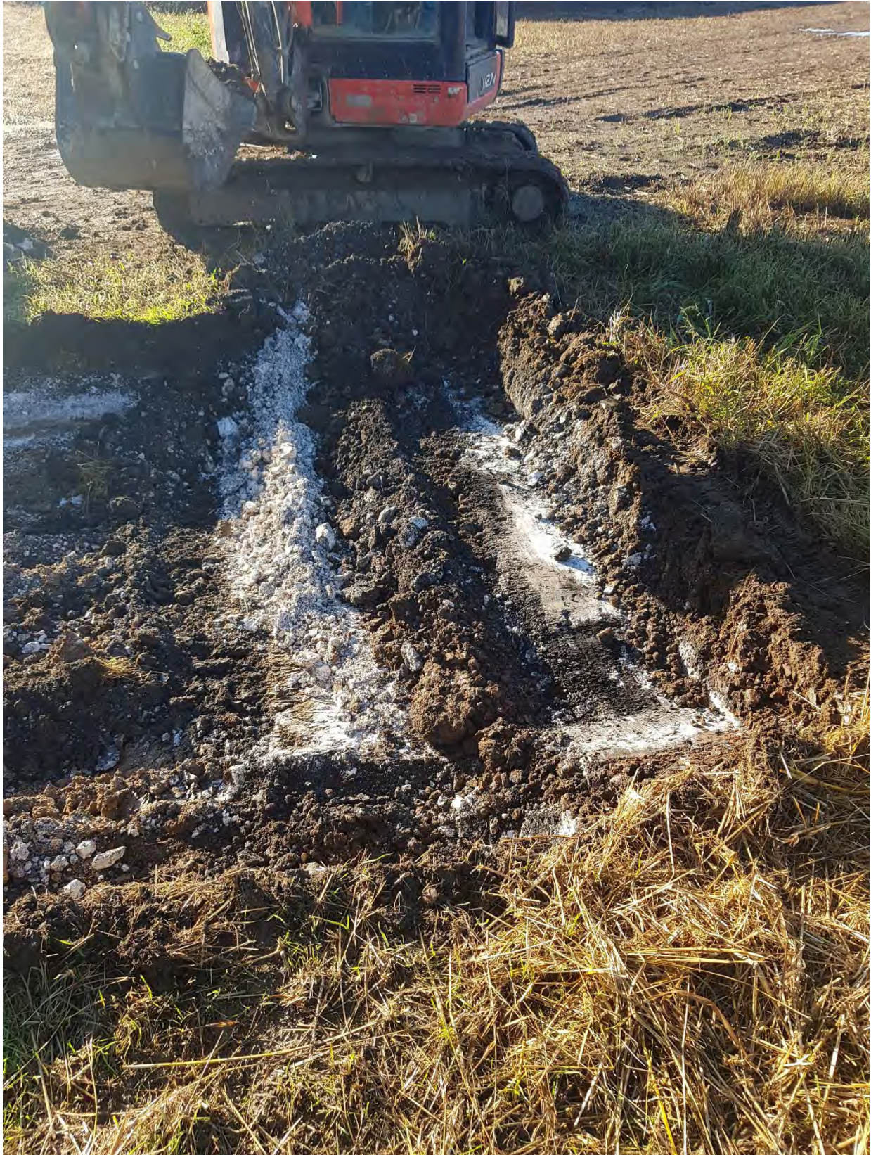
Plate 10 – View of excavation in progress
