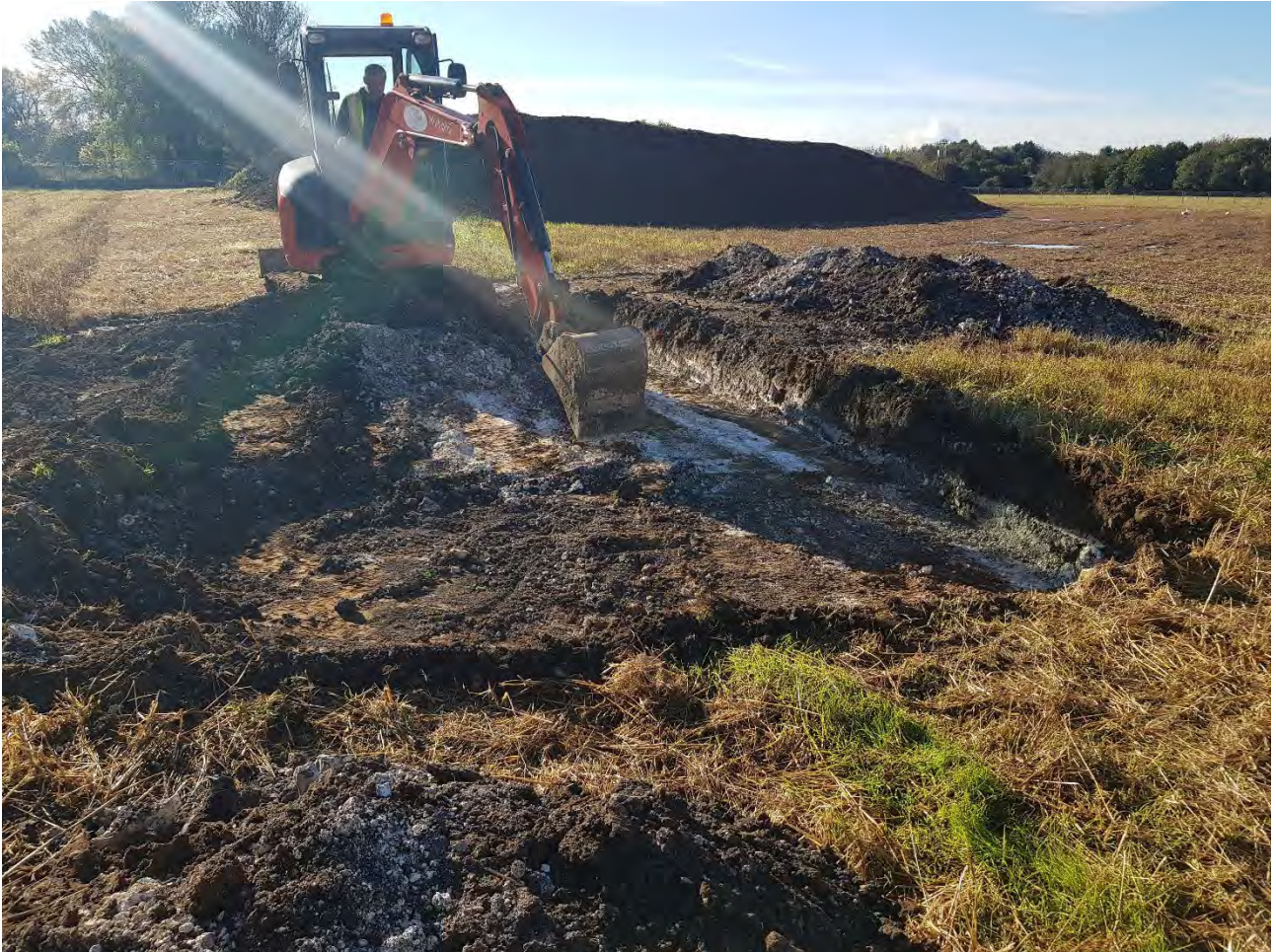
Plate 12 – View of excavation being extended in length
