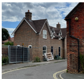
Pair of new-build houses under construction in The Twittens - these have upvc windows and doors.
