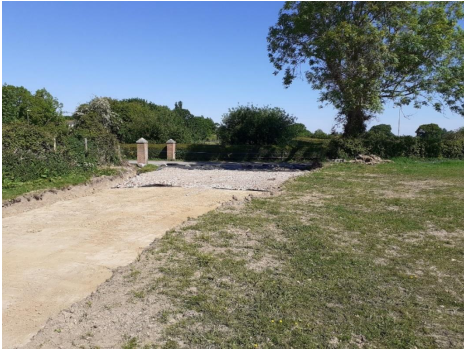
Photograph taken in May 2020. The bellmouth and first 30m section of the road is still a work in progress. Brick piers outside have now been removed.
