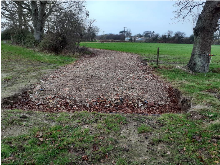
Photograph taken in December 2020 of the road built to date. This has been built to the south of the T15 oak tree on the southern side and is not yet complete. It remains 9.2m short of the boundary with the Woods Estate.
