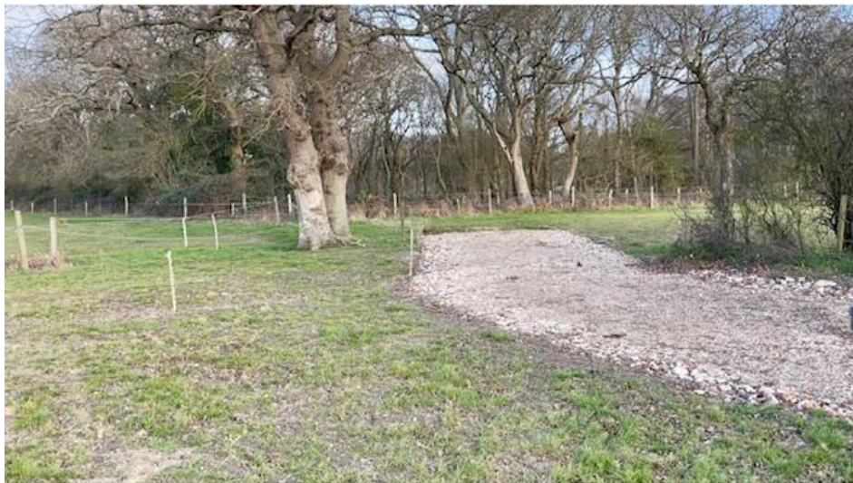
Photograph taken in March 2021 showing the road construction to date on the southern side of the T15 oak tree.
