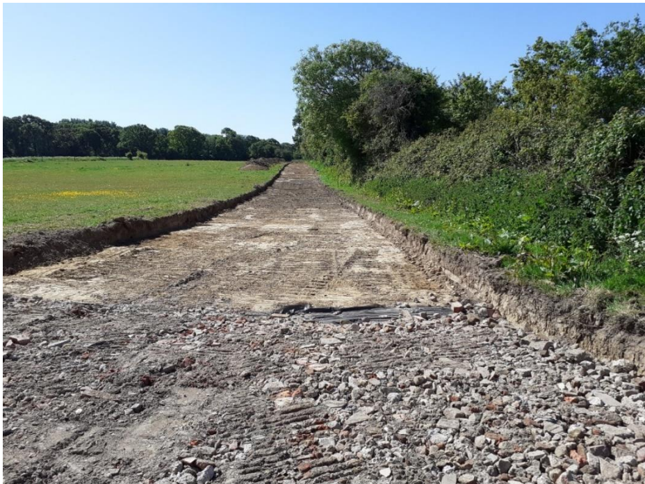
Photograph taken in May 2020 of straight alignment of road looking southwards from the entrance.
