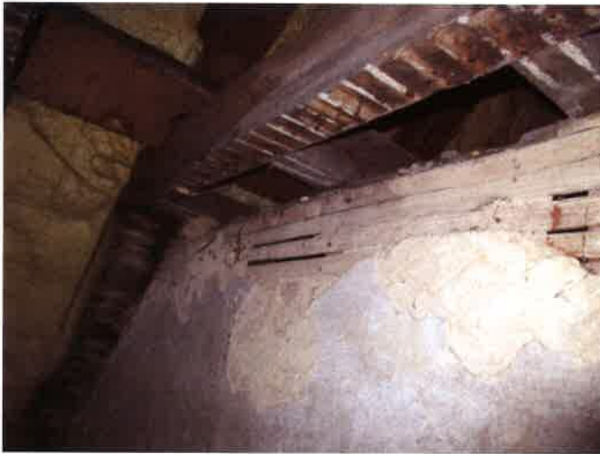
p 36 lath and plaster
