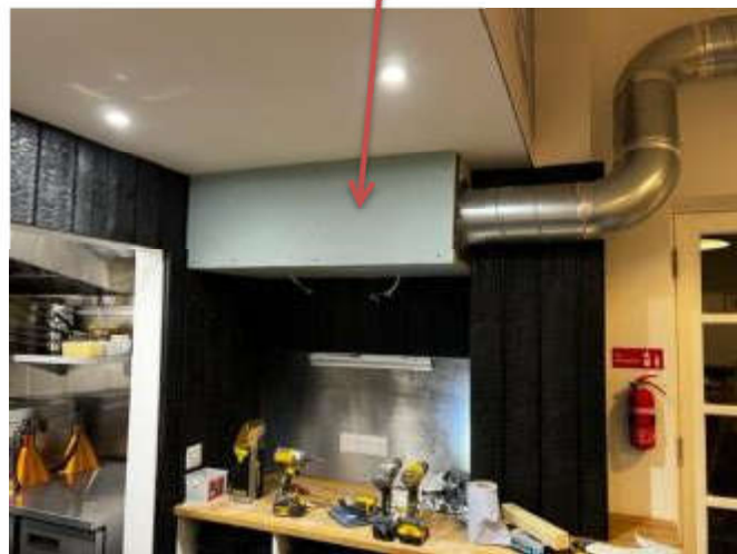
Boxed and sound proofed fan with access hatch for changing carbon filter
