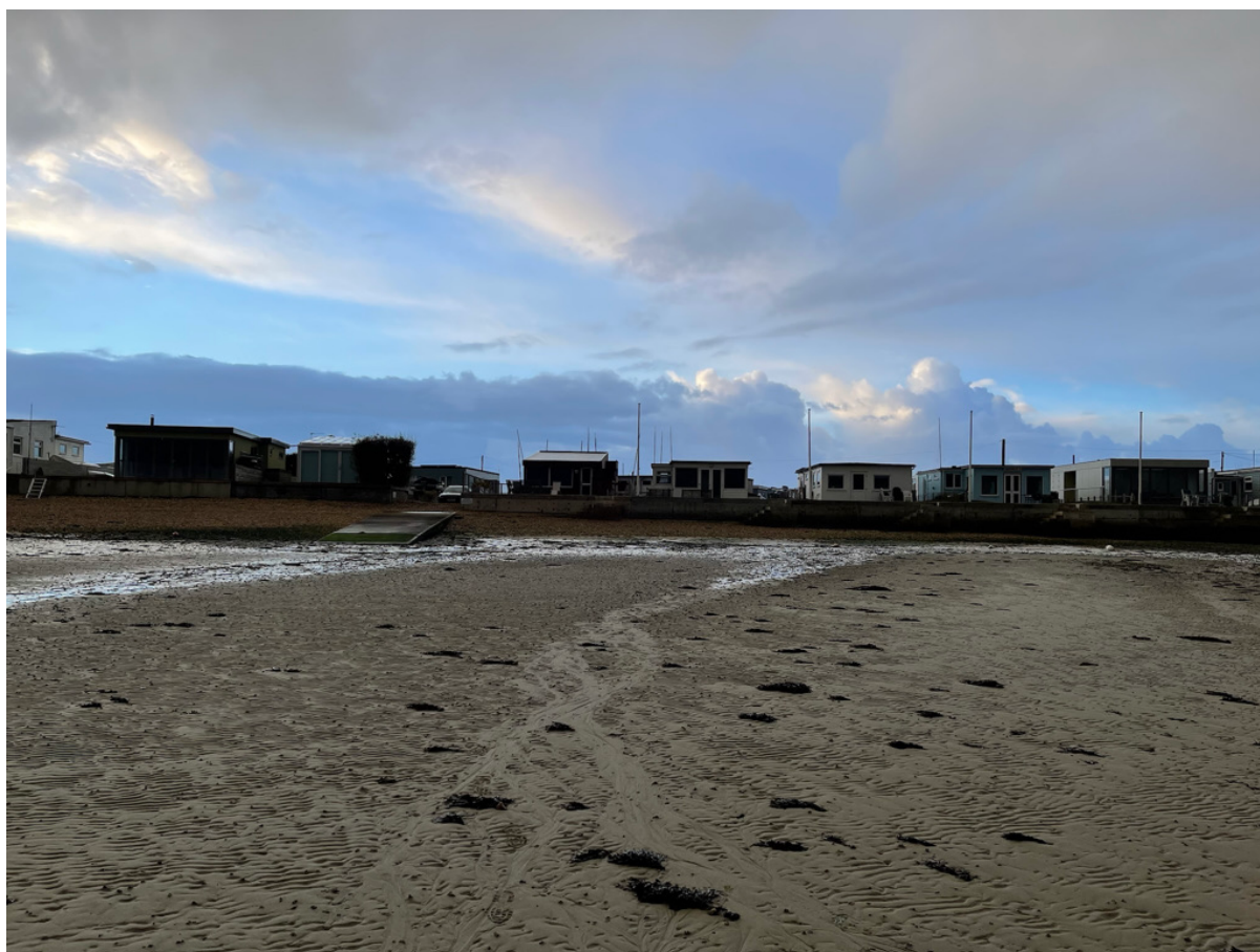
Photo 3: Looking south with new cladding, locker and strengthened sea wall. 22, The Kench is immediately to the right of the slipway.
