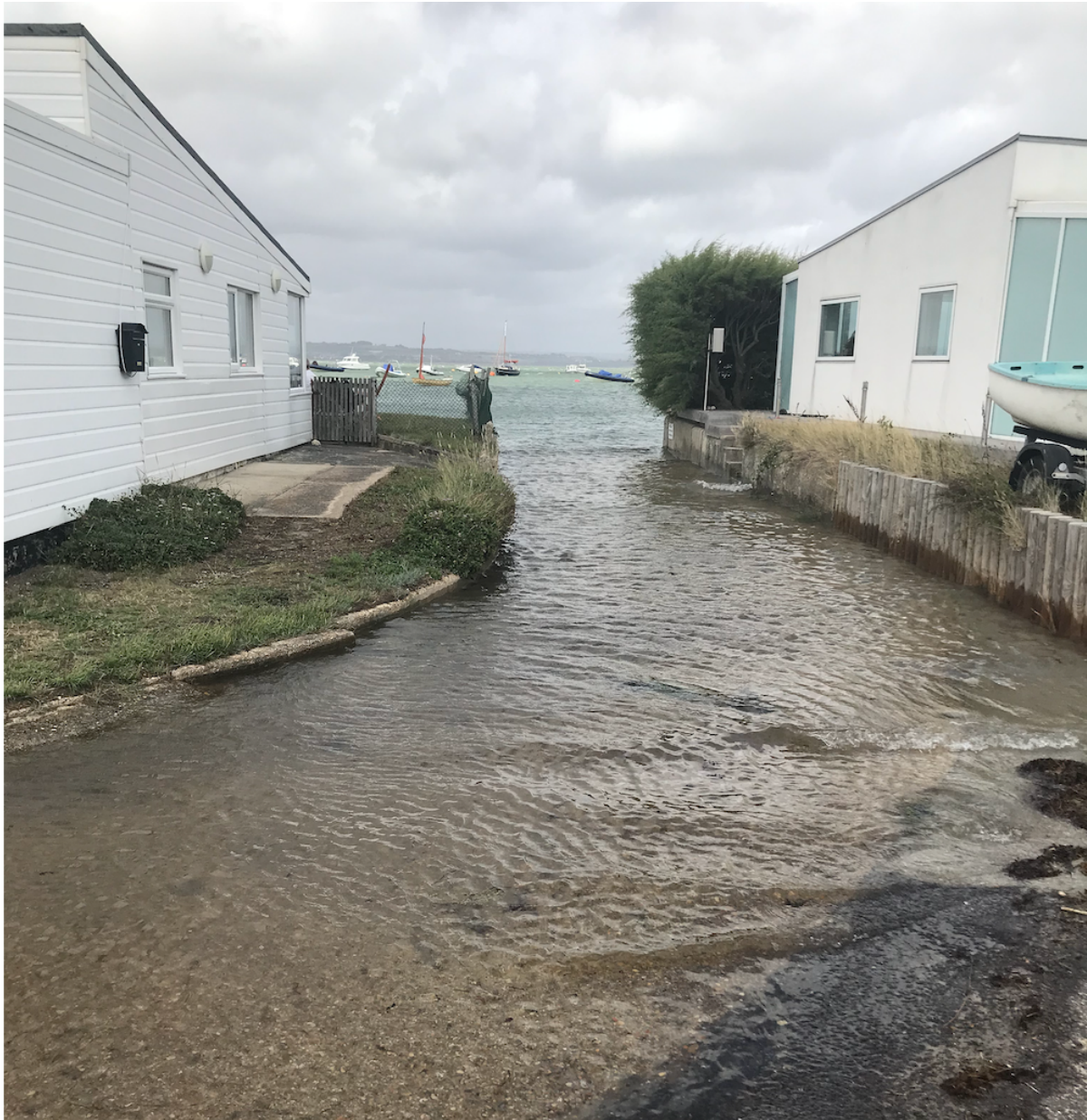
Photo 1: Looking north on a high tide with original white cladding
