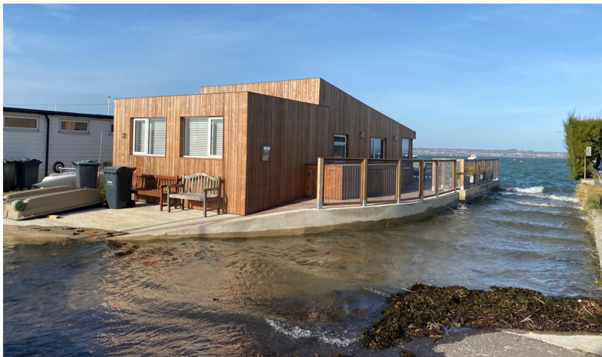
Photo 2: Looking north with new wooden cladding, locker and strengthened sea wall.
