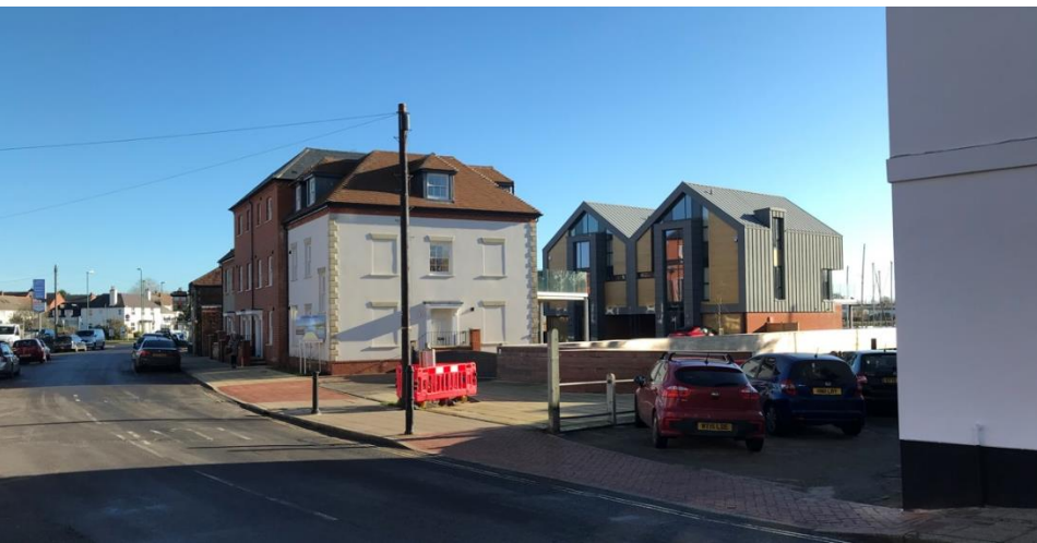
Figure 1 Application Site Viewed from the North-West
