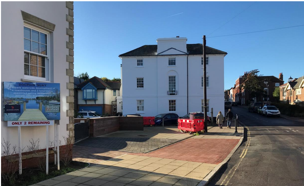
Figure 3 View West Across the Application Site – 29 Queen Street in Background
