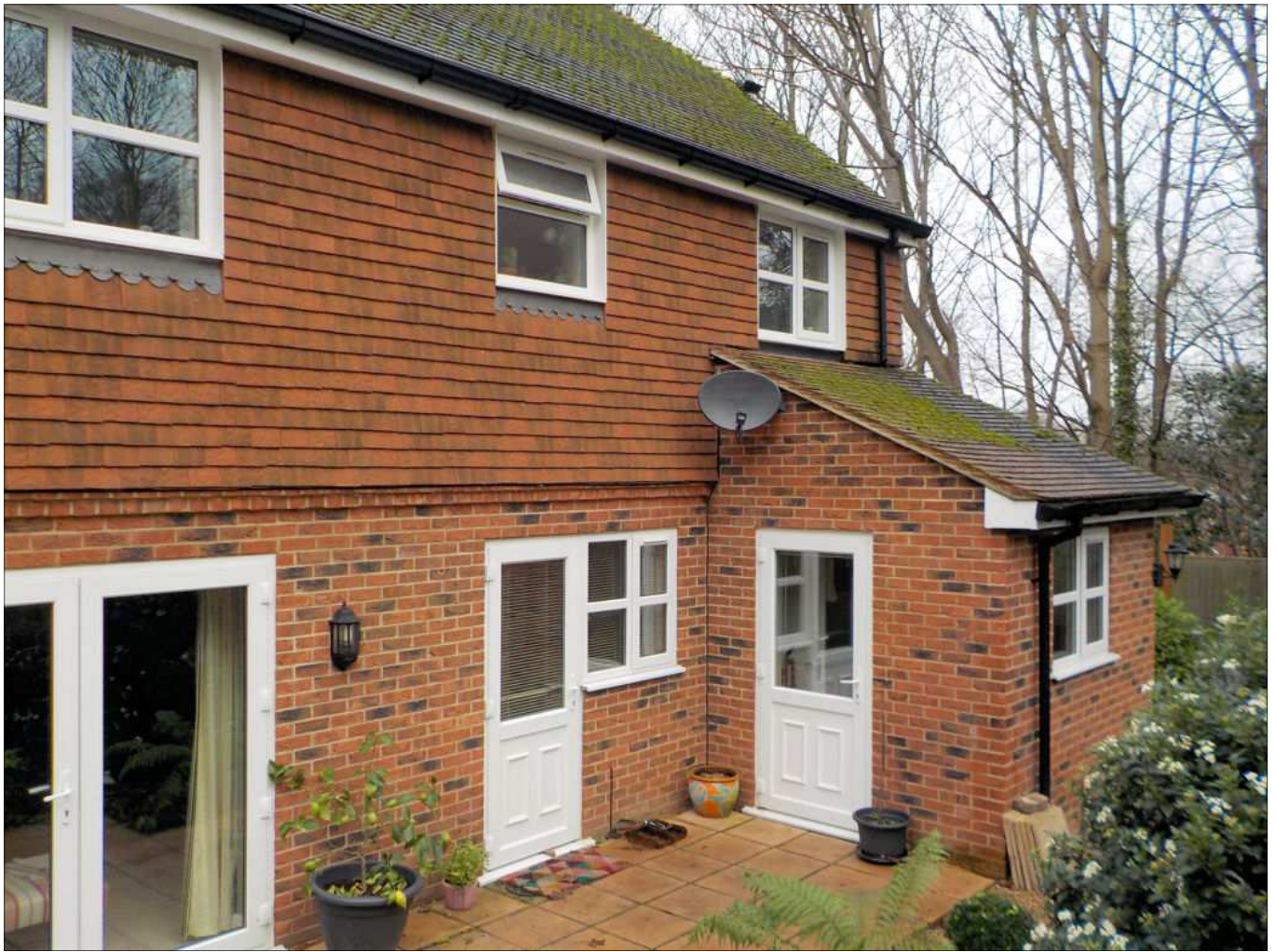
Rear of No. 2 Chace Gardens - location of extension
