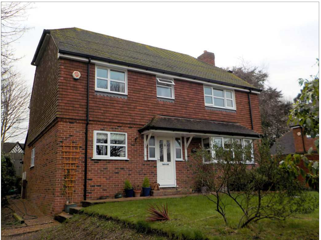
Front of No. 2 Chace Gardens
