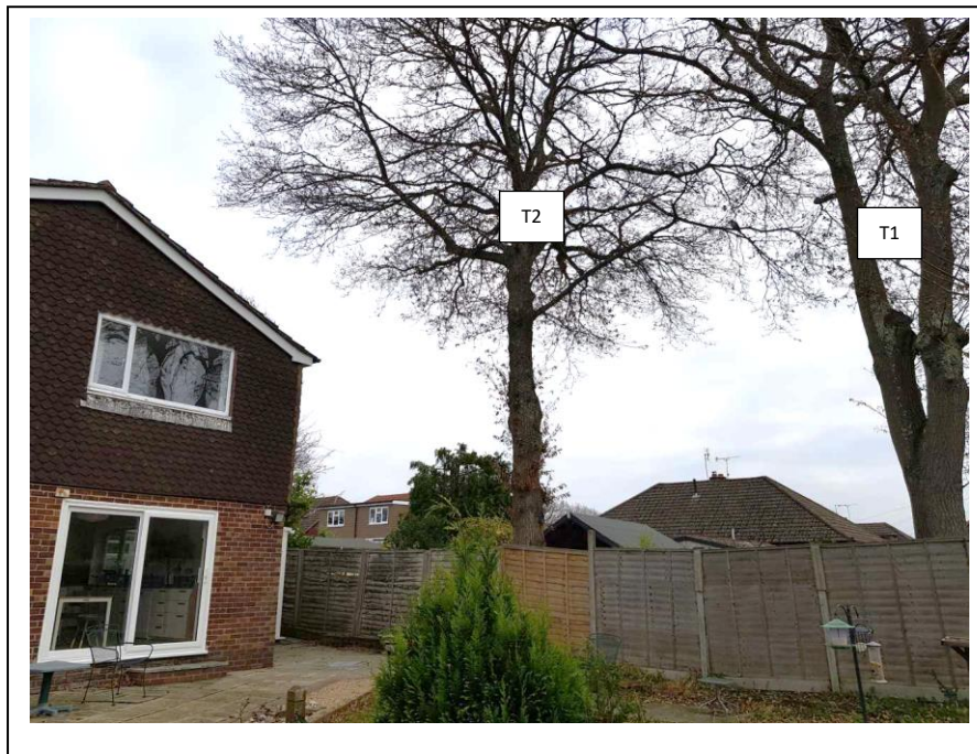
View of rear left corner of dwelling
