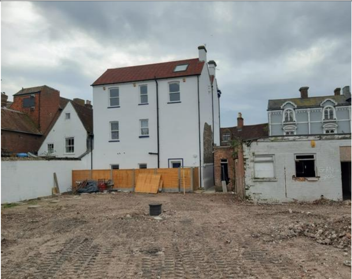
Figure 3: Rear elevation of 9 & 11 East Street.
