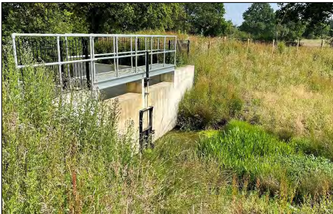
Figure 2-6: Flood attenuation area control structure (02/07/2021)
