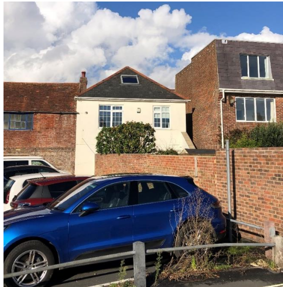
Figure 9: Rear Elevation from South Street Car Park – South
