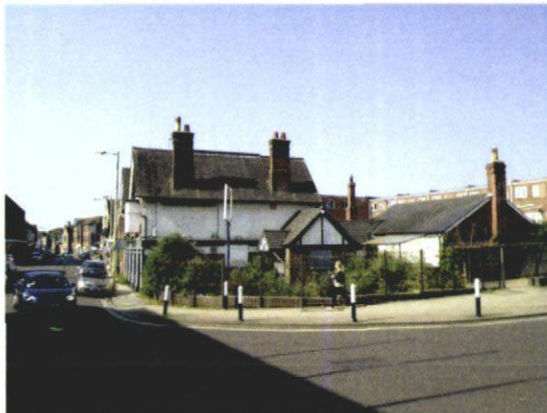
Current Public House site on corner of access road
