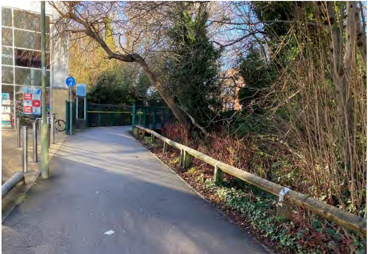
Image 3.12: Photograph of NCN Route 22 continuing into Havant Town Centre
