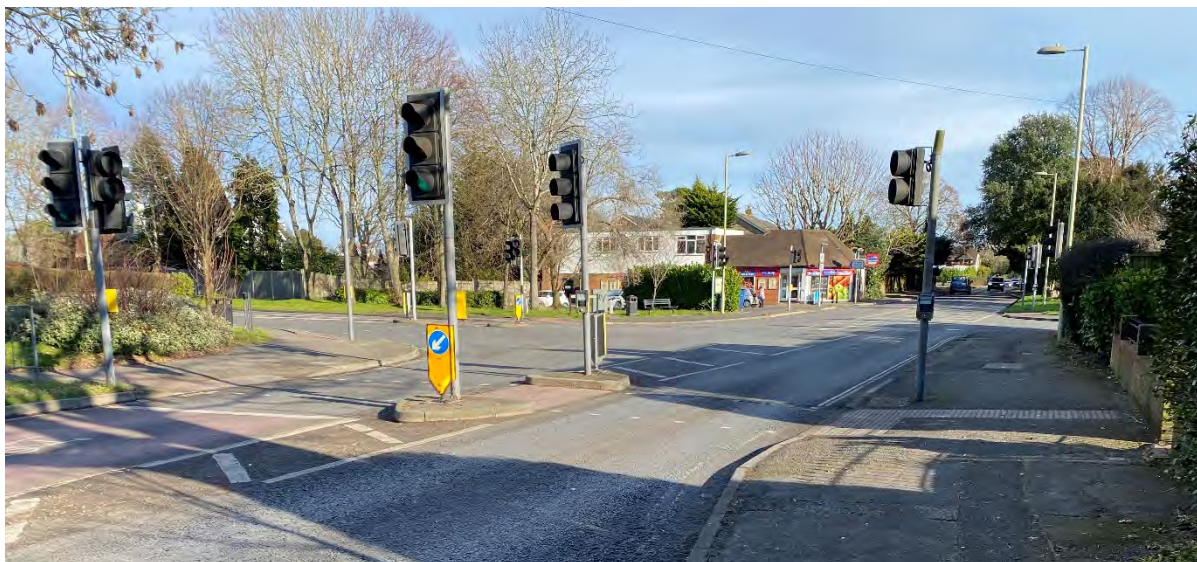
Image 2.8: Photograph of Signalised Crossing Across Emsworth Road
