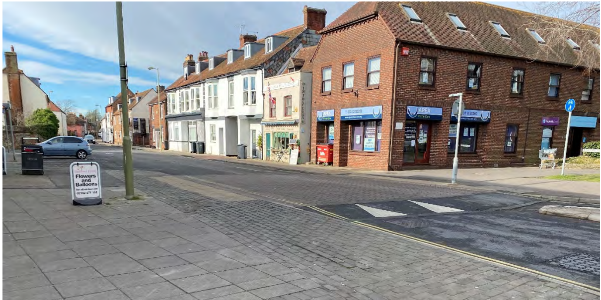
Image 2.2: Photograph of Raised Crossing Across West Street adjacent to Park Road South
