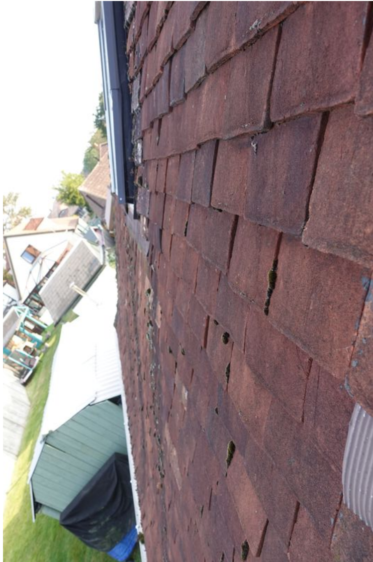
Plate 2: Eastern roof aspect
