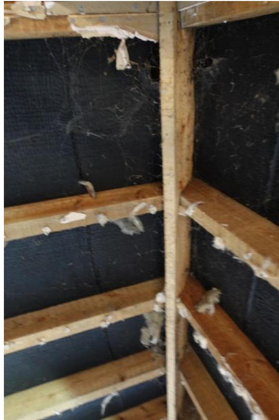
Plate 5: Supporting timber beams and cobwebs
