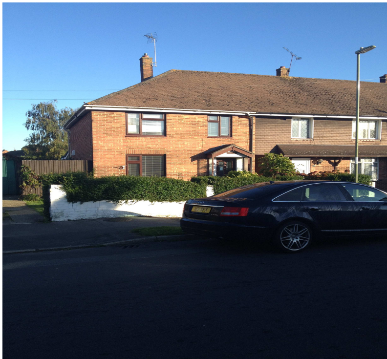
View of the existing terrace looking east
