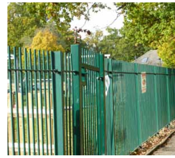
Figure 31: Vertical bar fencing for school boundary
