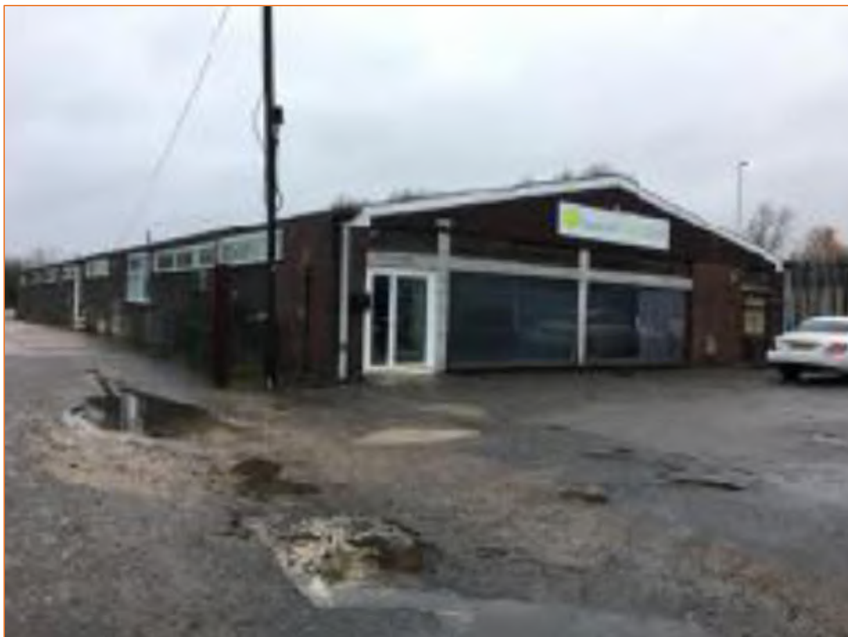
Figure 3: South and East Elevations of Existing Building (Source: Lowans Ecology & Associates)
