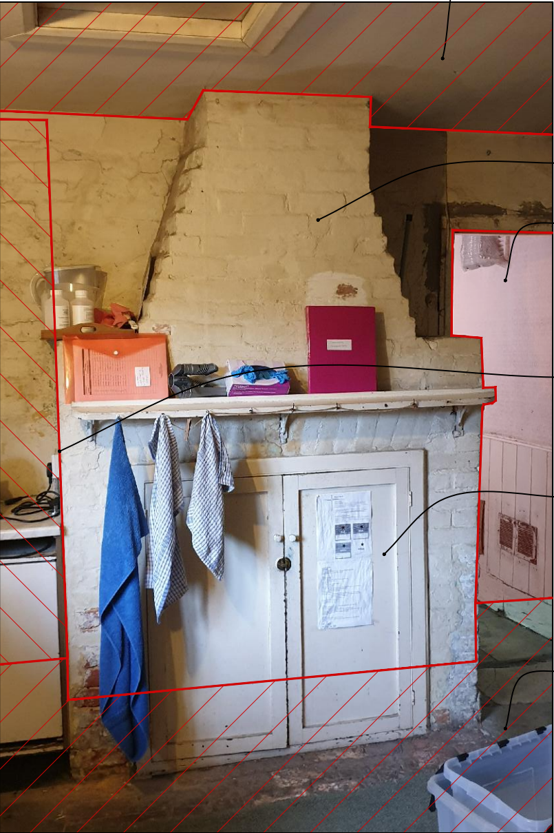
Chimney Breast within Staff Kitchen / Storage Area
