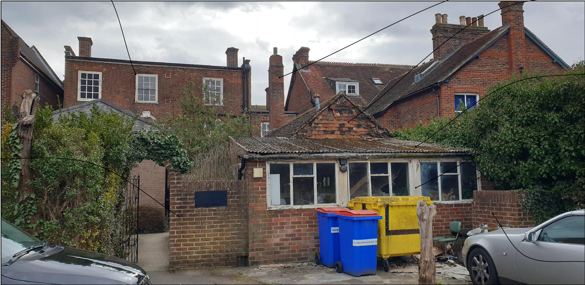
Rear South Elevation as viewed from Car Park
