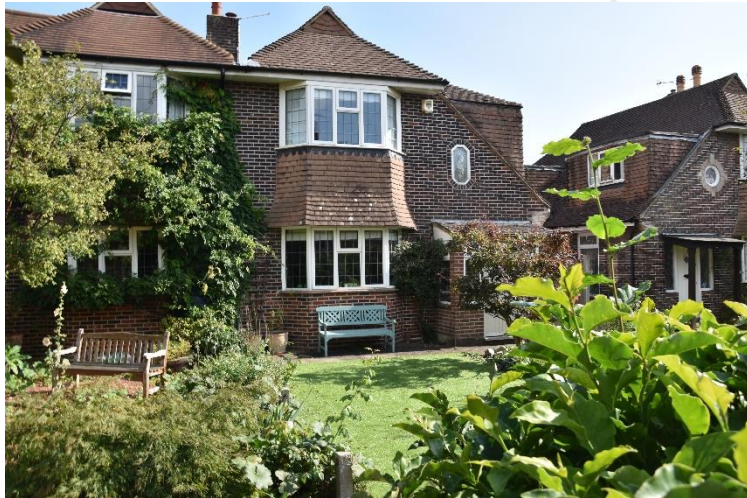
The earlier houses opposite no. 26 feature a higher level of detailing
