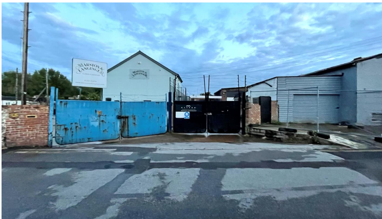
Gated Accesses Serving Units W1/W4 and 6/W2
