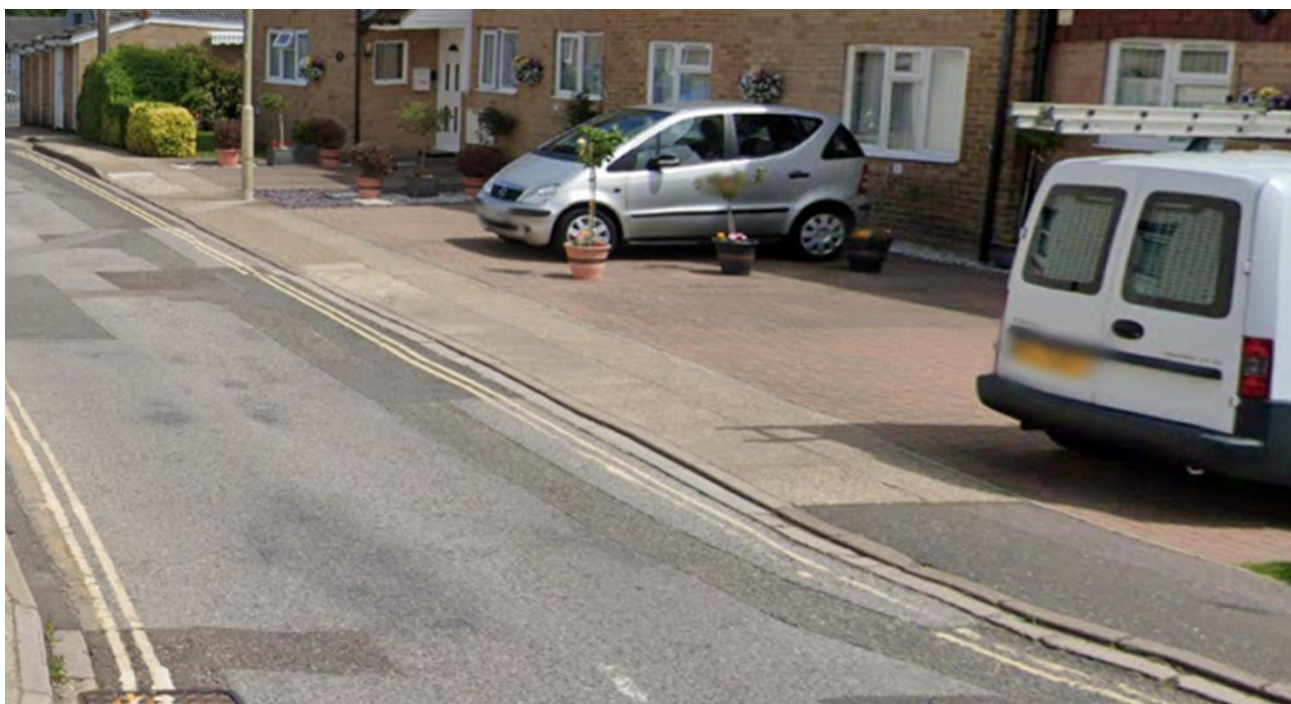
Figure 2.6: Existing Footway on Seagull Lane
