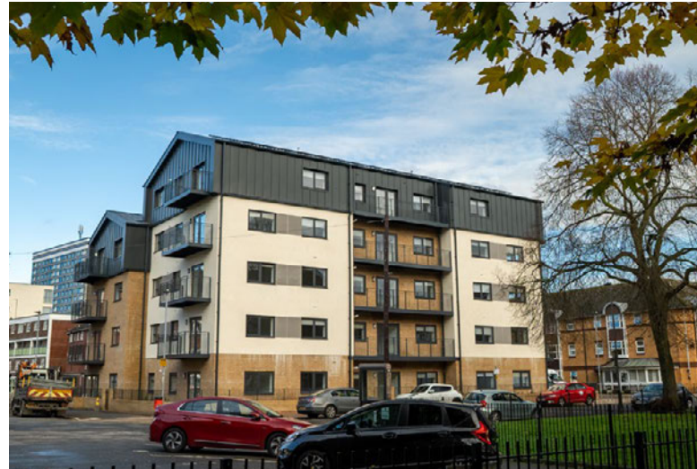
PCC development - Albion House, Portsmouth.
