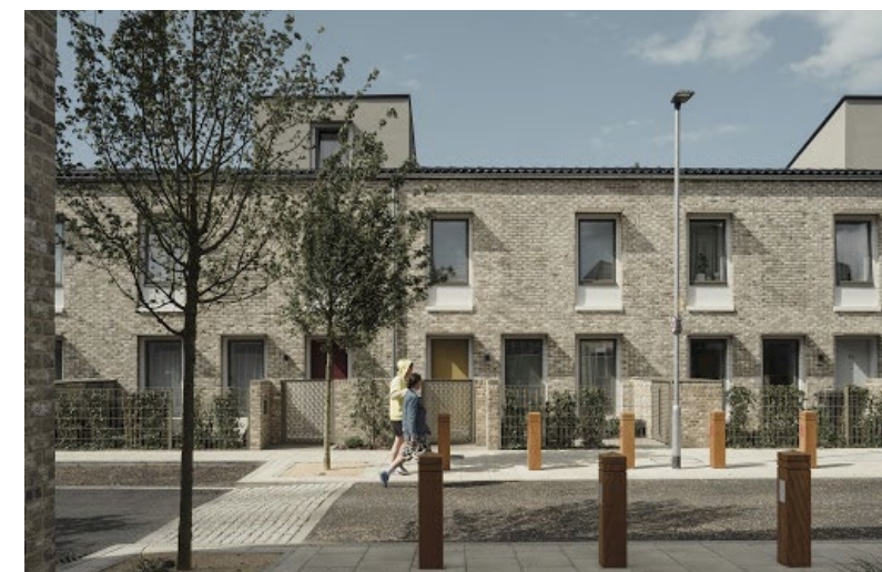
Goldsmith Street, Norwich, source: Mikhail Riches
