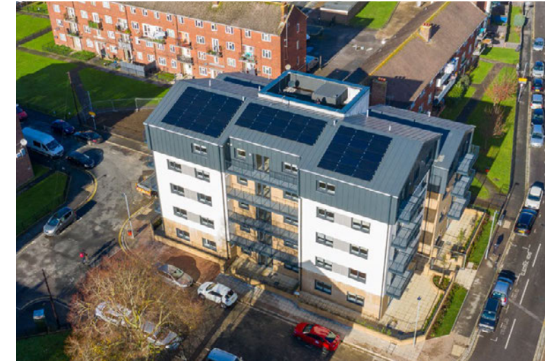
PCC development - Albion House, Portsmouth.
