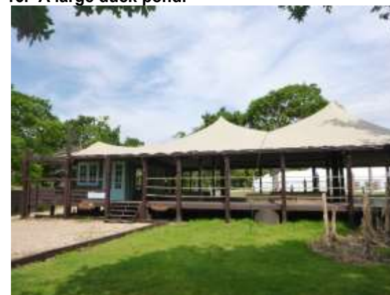
18. The decking and canopy to the south of the marquee.
