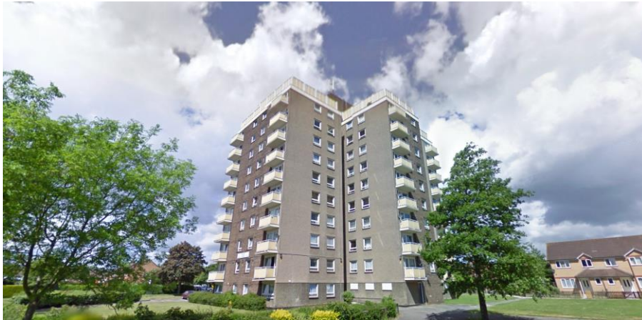
Existing view of Solent House from the associated car parking area
