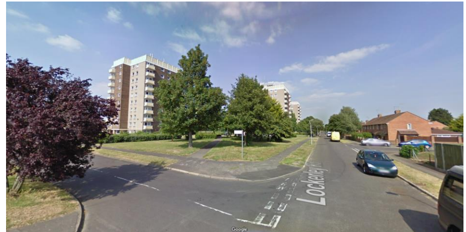
Entrance to Swarraton Road from Lockerley Road [Google Maps]
