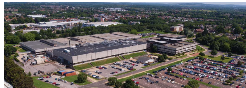
AERIAL VIEW – NORTH EAST
