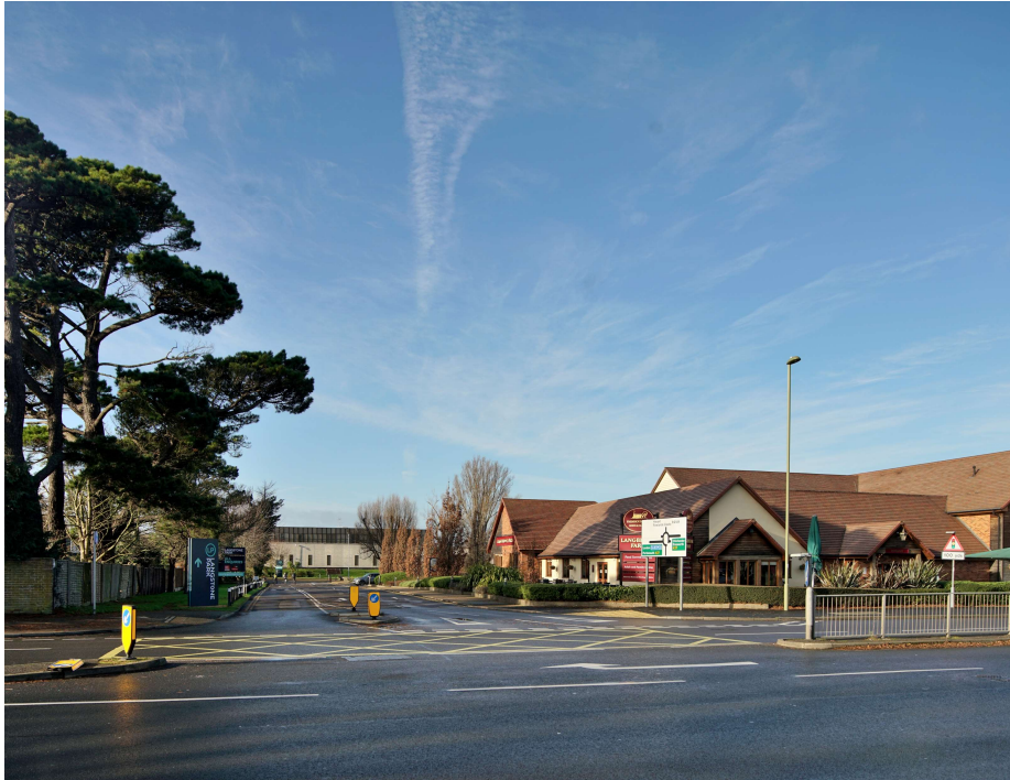
EXISTING VIEW OF LANGSTONE ROAD SITE ENTRANCE
