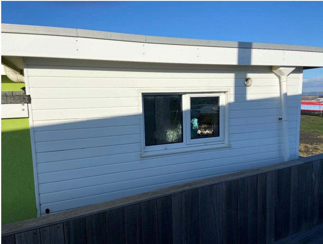
Part elevation of pvc clad
