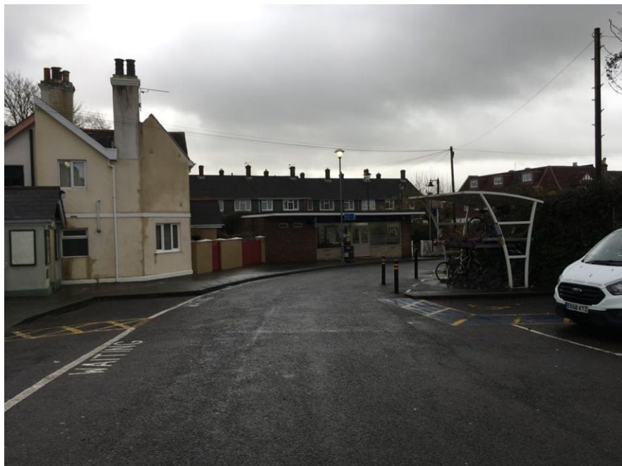
Figure 2: Station access road looking towards North Street
