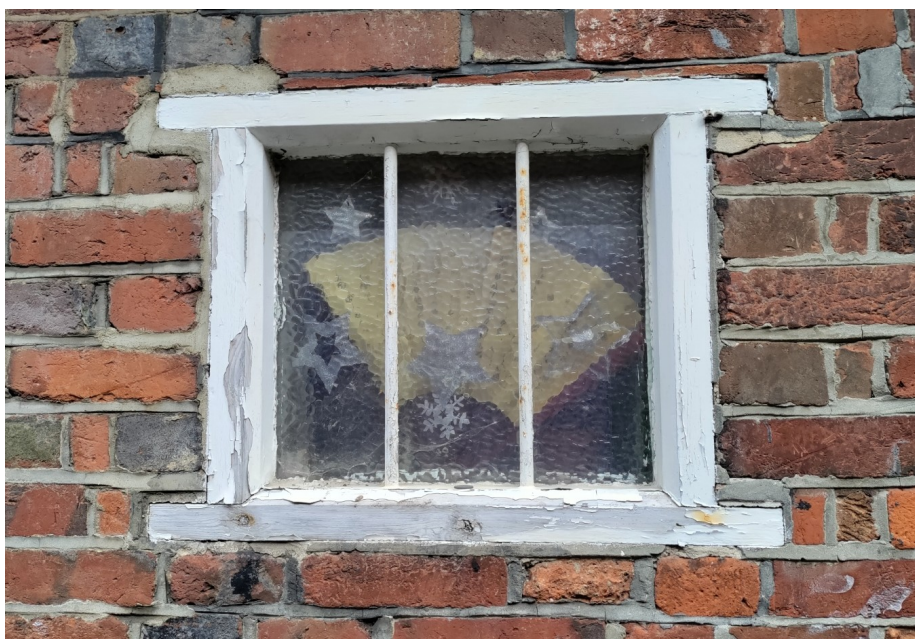
Figure 2: Historical window; due for surface paint removal, treatment and repainting to conserve. The visible decals are temporary and are adhered with water for removal without marking.
