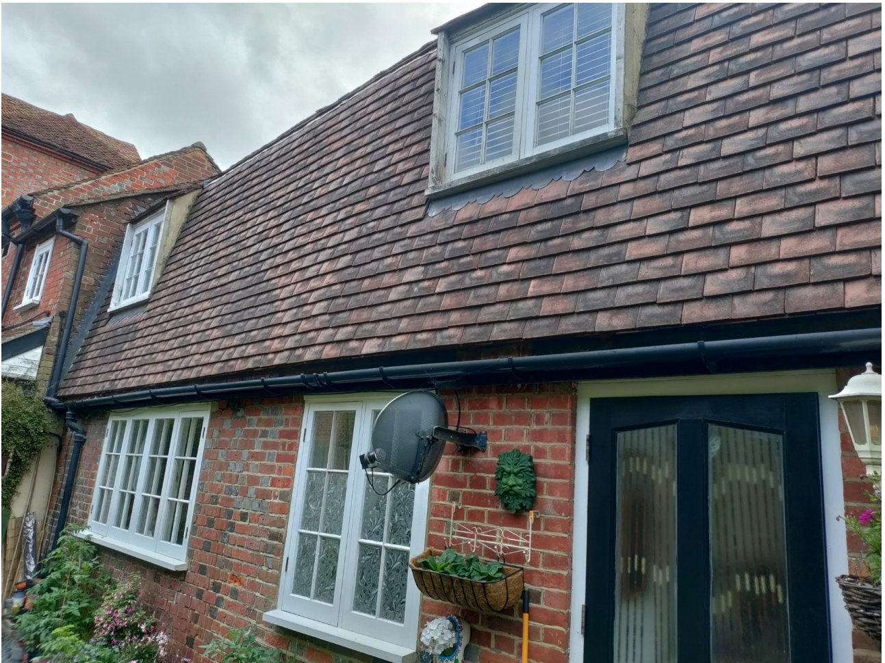
Figure 4: All East-facing windows. On the bottom, the living room window and the utility/toilet window with removable privacy film. Above the 2 nd and 1 st bedroom windows.
