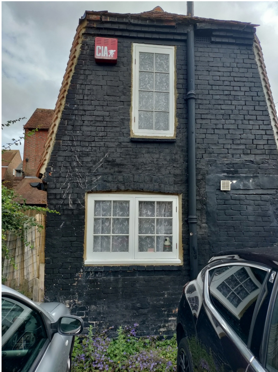
Figure 3: North aspect of 5 Elmore Court. The main building of 21 East street can be seen in the background. The lower window is the kitchen and the upper, main bedroom.
