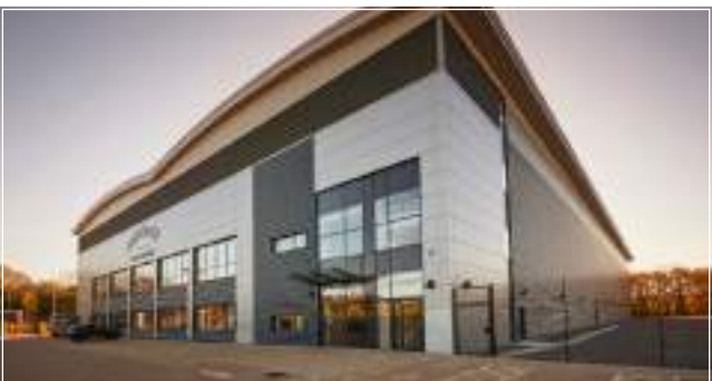
7 Close up view of existing Fat Face build
