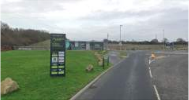
1 View from Dunsbury Park Entrance Route
