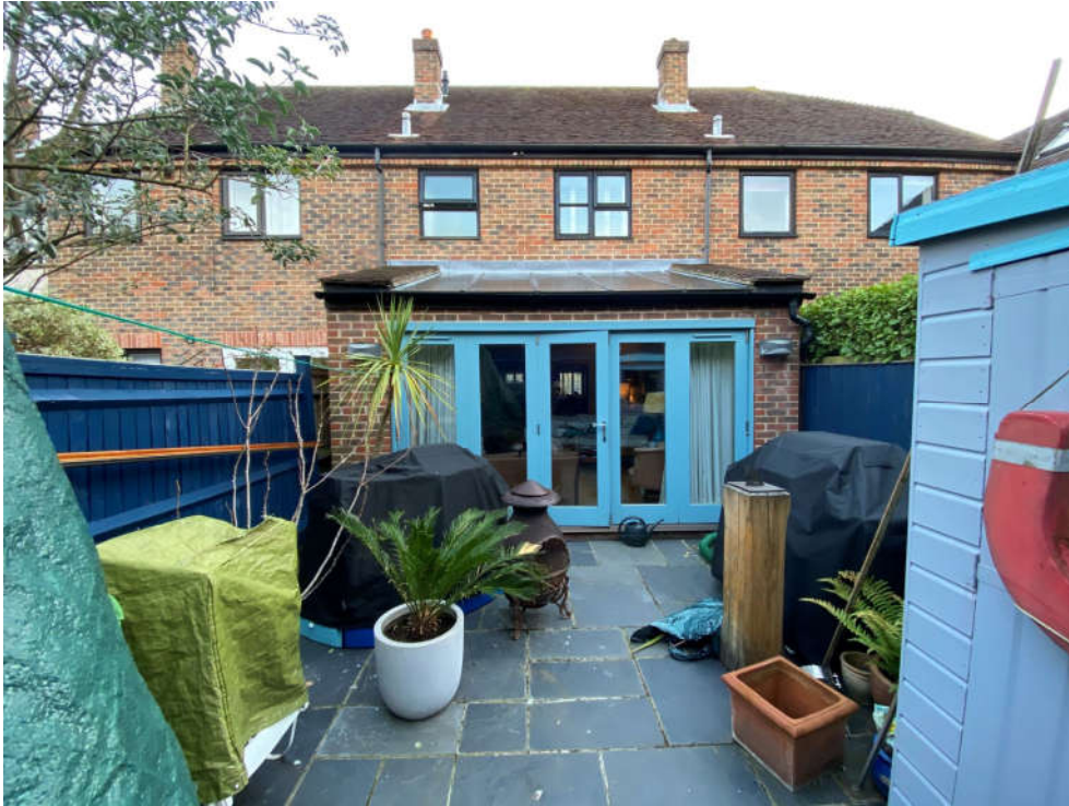
Existing rear elevation of dwelling.
