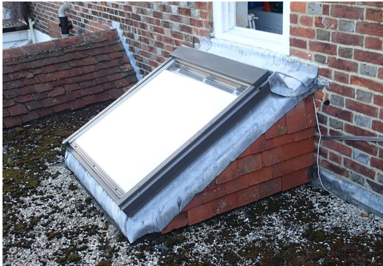
Figure 7: Existing Rooflight to hallway.
