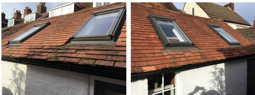
Figures 5 & 6: Existing Rooflights to Kitchen.
