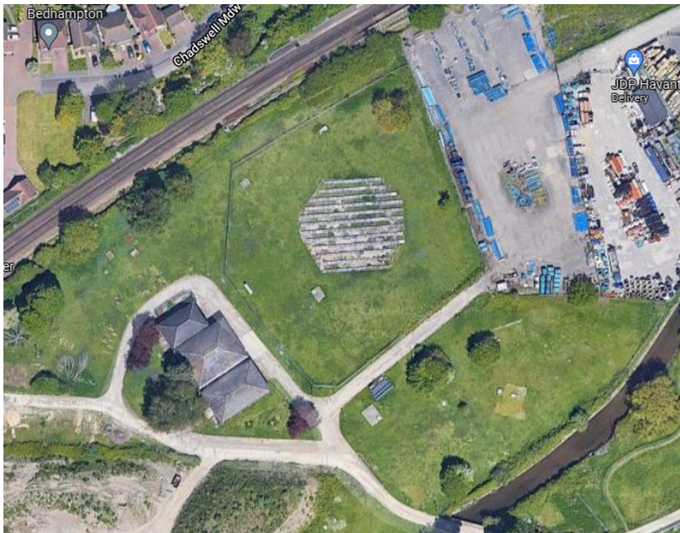
Figure 1: An aerial of the site showing the existing solar panels.
