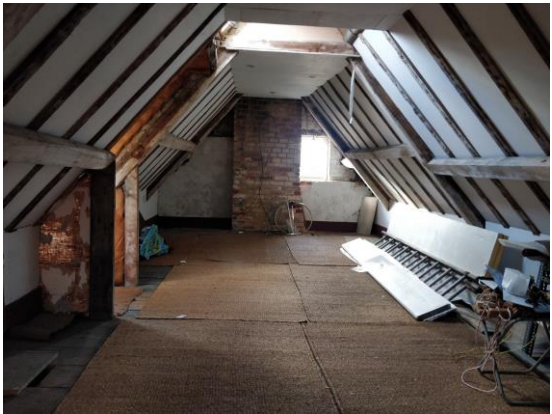
Roof Space [North]
