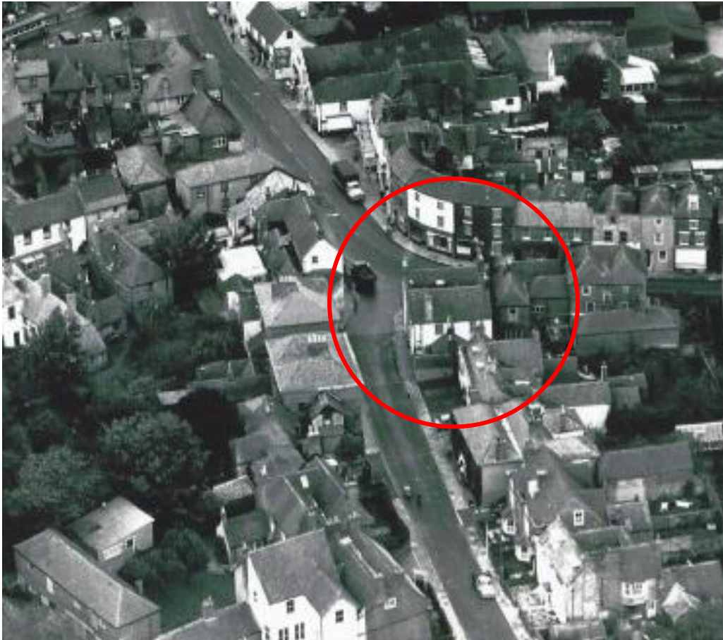
Aerial photograph 1961 – Includes rear extension and outbuilding
