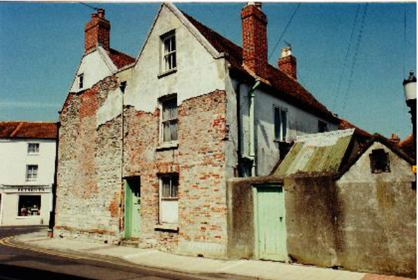
Rear Extension with corrugated roof. Date unknown.
