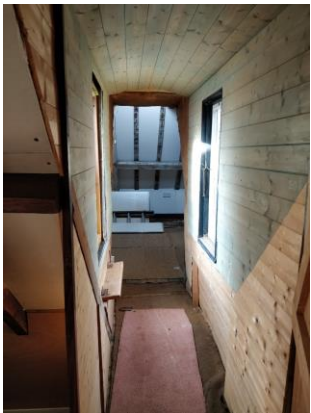
Access through roof spaces
