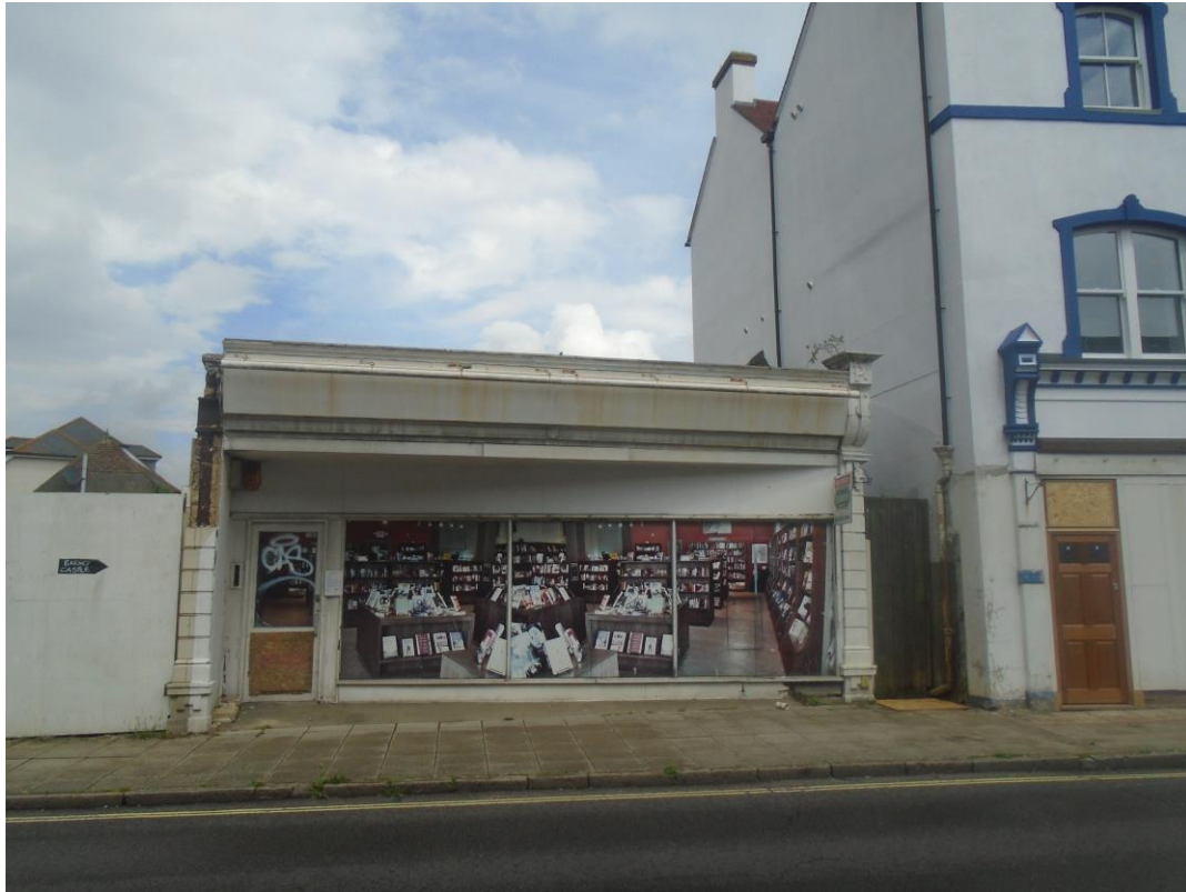
Figure 1. Empty shop unit.
