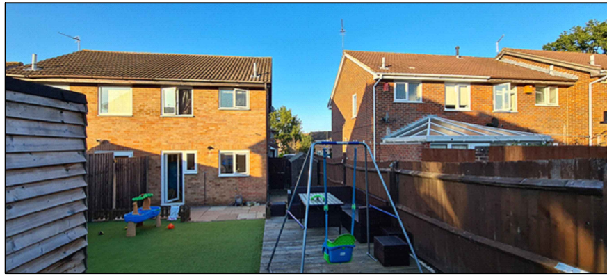
EXISTING PHOTO REAR ELEVATION
