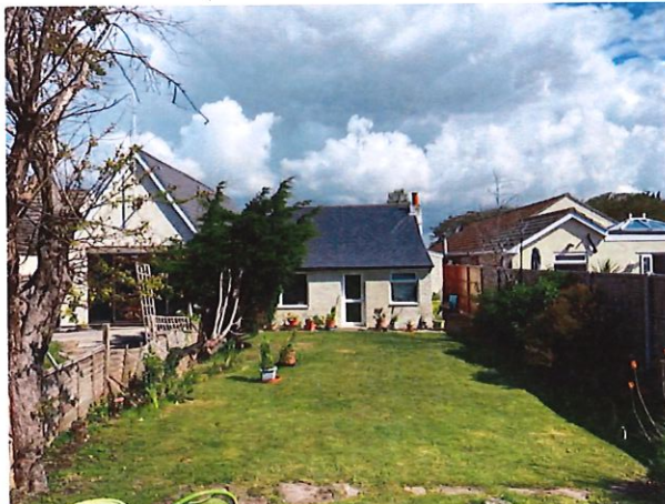
The rear (south) elevation of the existing bungalow, and that of neighbours.
