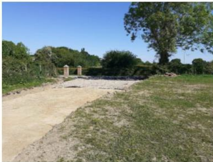
Photograph of existing Ash tree adjoining Tournurbury Lane, to be retained
