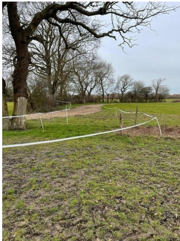
Photographs taken in March 2021 of the pegging out of approved road alignment (APP/17/00207) past the T15 oak tree from both directions. The road route in this direction would be too close to overhanging branches.
