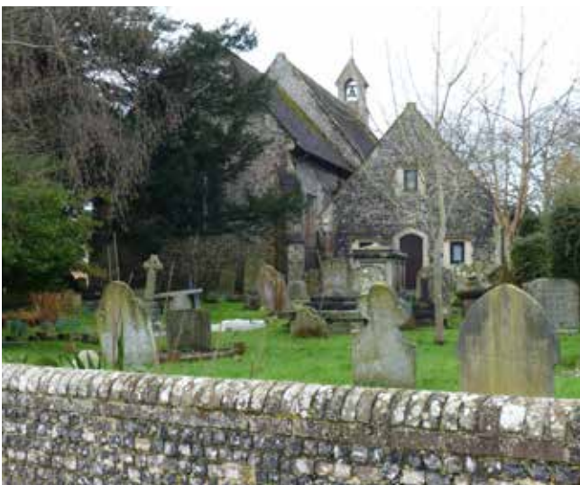
The listed grade two Church of St Thomas dates back to the 12th century (grade II)
