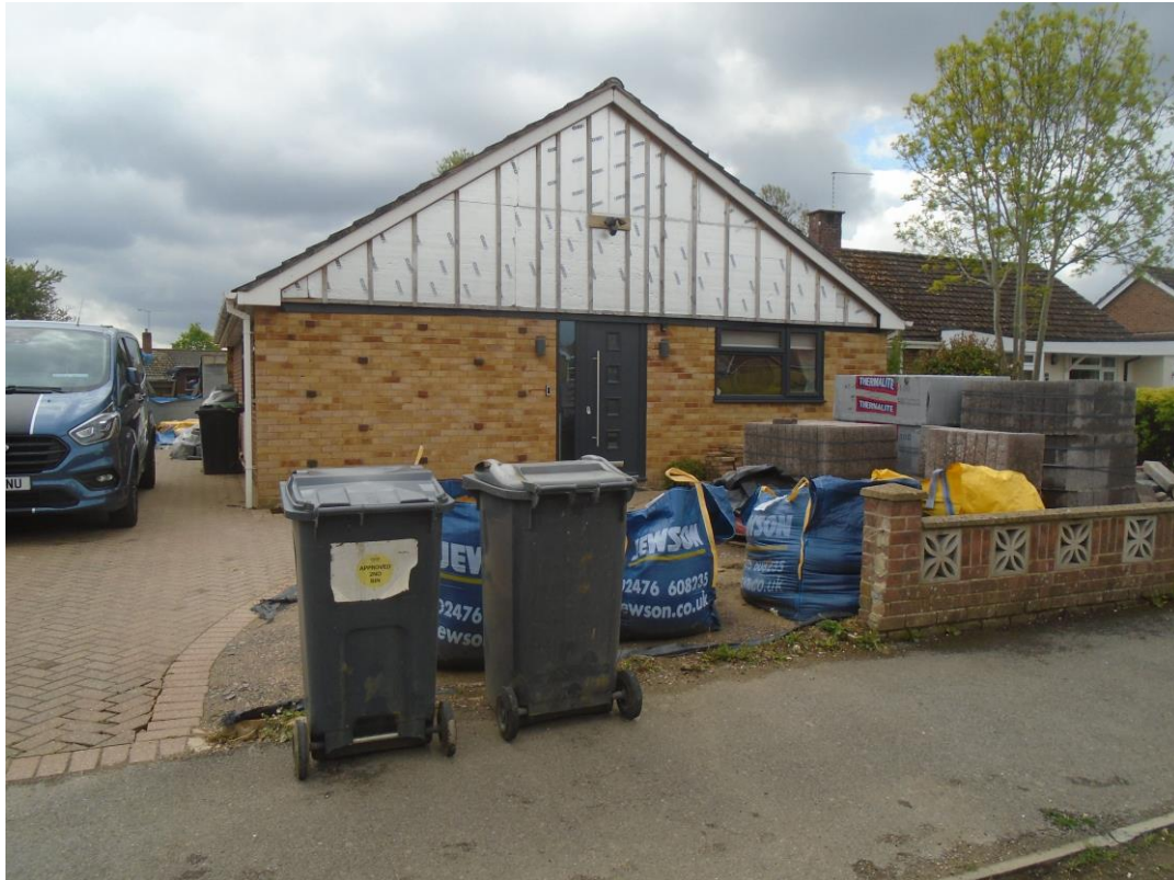
Figure 1. The frontage of the dwelling to Spring Garden.
