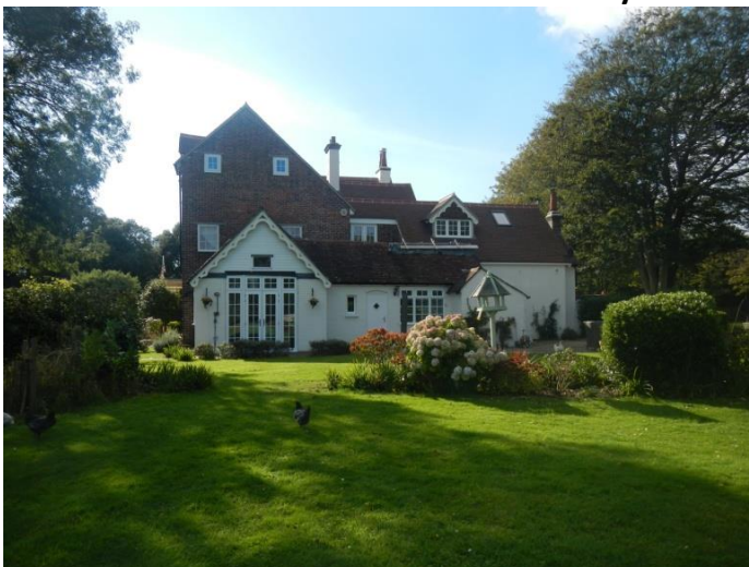
East elevation, single storey structures
