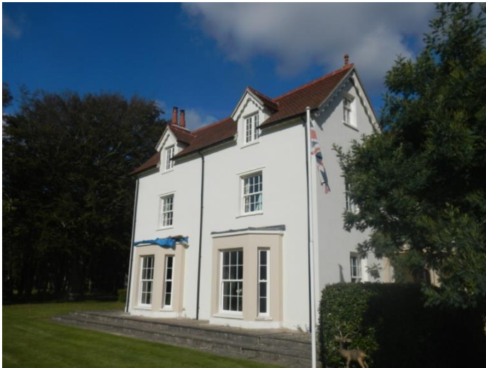
S elevation (unaffected by works)
