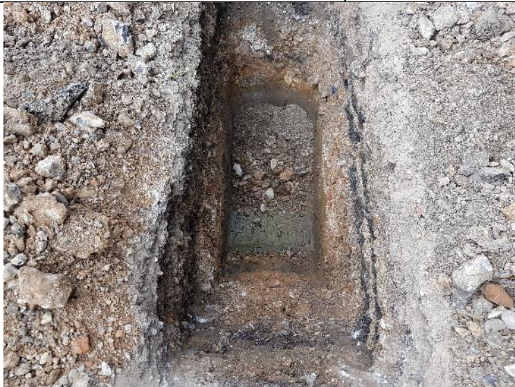
Plate 7 – TP04 – Trial pit
