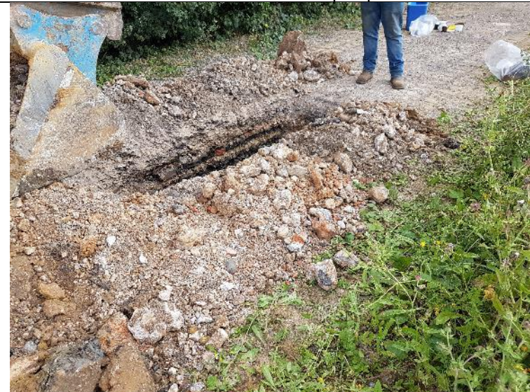
Plate 8 – TP04 – Trial pit spoil
