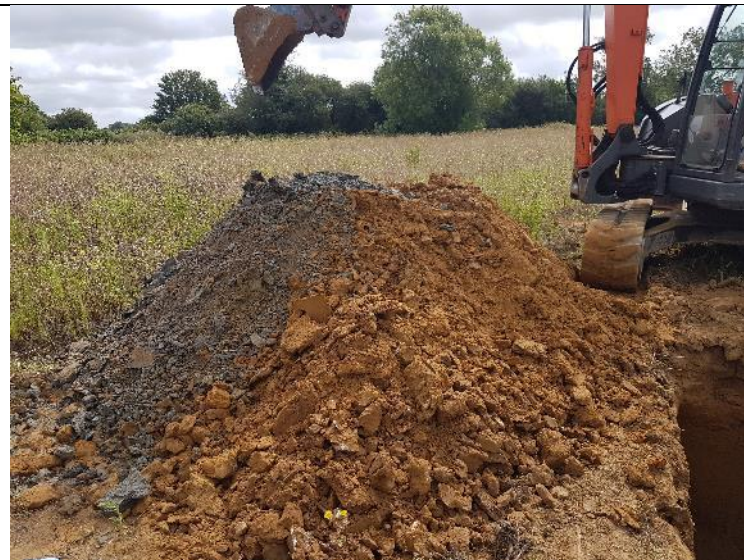
Plate 2 – TP01 – Trial pit spoil
