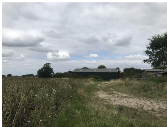
Photograph 2. On-site building and access track.
