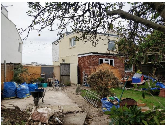
Figure 4: Rear of existing property
