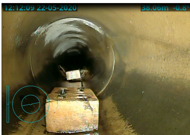
Bricks found in the pipework
