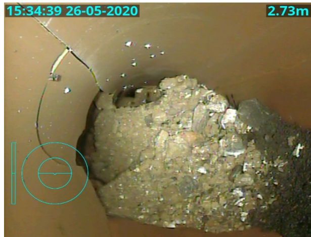
Pipework shows rear access BLOCKED
