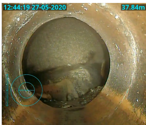
PARTIAL FLOOD (STATIC WATER)
