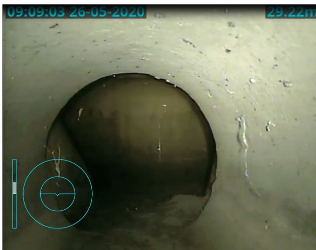
Pipework CLEAR, has cracking laterally but no displacement
