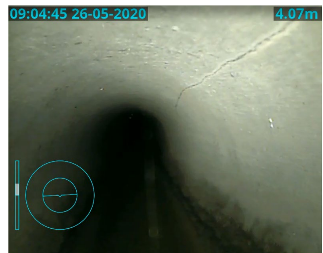
Pipework CLEAR, has cracking laterally but no displacement
