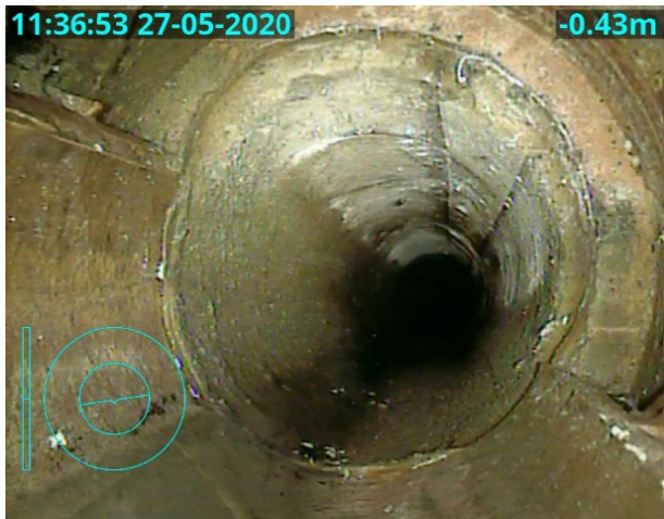
BROKEN JOINT – PIPE RUNS CLEAR
