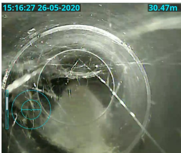
Pipework shows LIGHT DEBRIS
