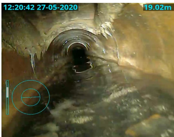
PARTIAL FLOOD (STATIC WATER)
