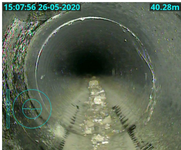
Pipework shows LIGHT DEBRIS
