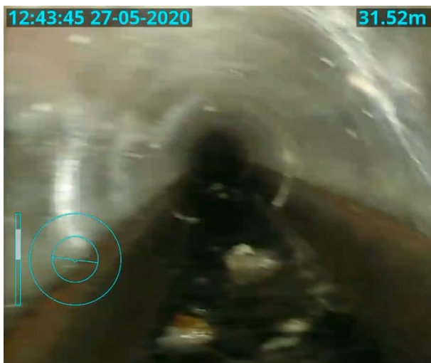
PARTIAL FLOOD (STATIC WATER)
