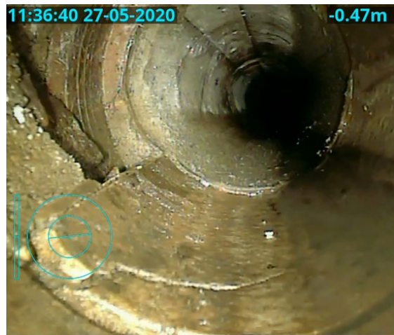
BROKEN JOINT – PIPE RUNS CLEAR
