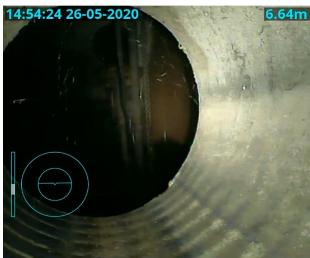
Pipework shows areas of POTENTIAL BLOCKAGE otherwise clear (or light silt)
