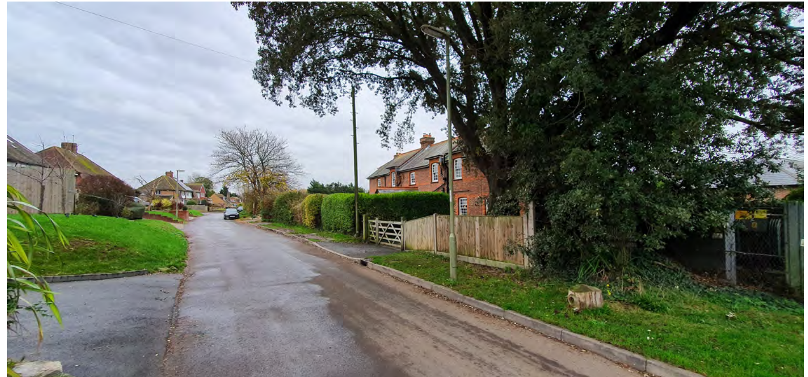
B View along Lower Road from outside Old Manor Farm
