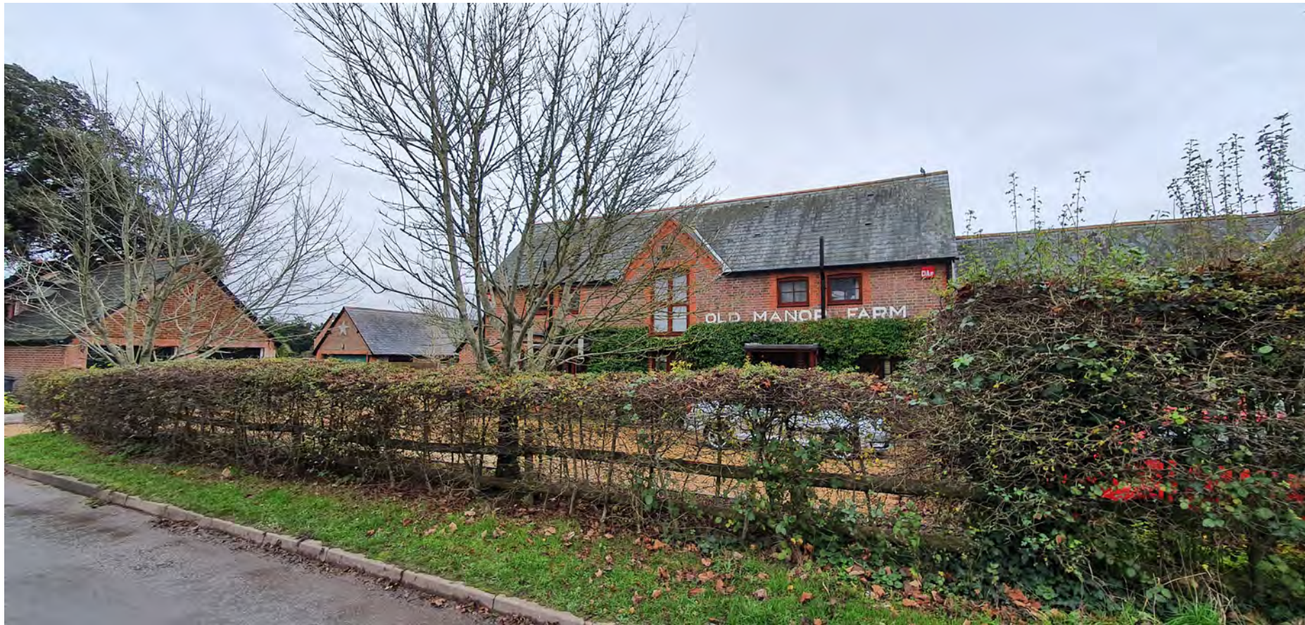
A Old Manor Farm - front view
